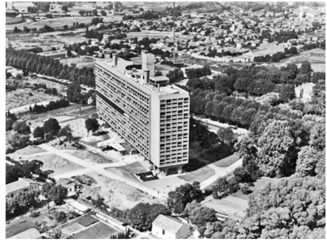
Fig. 6.8 Le Corbusier's Unité d'habitation, Marseille, France, 1945–52. Designed as a small, self-sufficient 'vertical town' for 1600 inhabitants, raised above the ground
