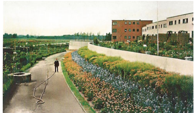
Fig. 25.5 Ernst May and Leberecht Migge (landscape architect), Römerstadt, Nidda Valley, Frankfurt am Main, 1929
