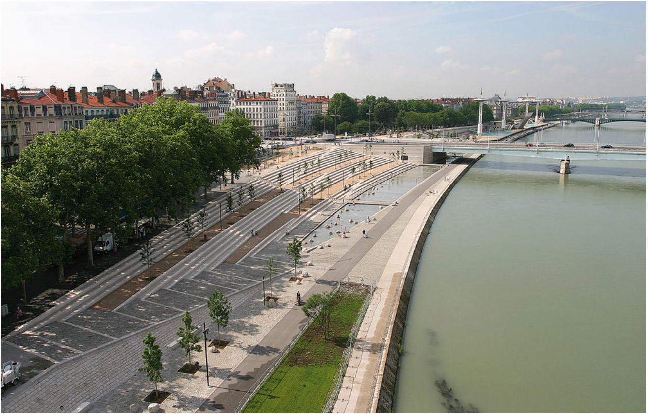
Fig. 13.8 Renovation of the right bank of the river Garonne, Bordeaux, 2015
