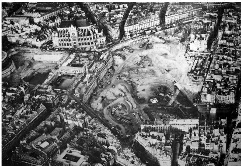
Fig. 12.2 Paris, the ‘Battle of Les Halles’: Urban void after demolition, 1973
