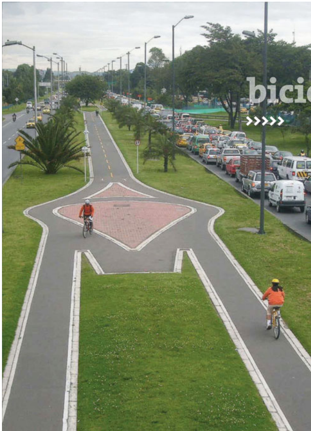
Fig. 22.6 Cycle lane in Bogotá, Colombia. Next to Sao Paulo, Bogotá has the largest network of exclusive cycle lanes in any Latin American city, implemented at the end of the nineties, and now covering over 350 km. Bogotá is also known for its intensive use of public transport, which has drastically reduced the number of cars, traffic and pollution. Transmilenio, the massive transport system in Bogotá and Soacha, is a system of rapid transit buses (BRT) in a closed type corridor system, branch-fed, with a raised platform and capsule stops where the fare is paid before boarding. Since it was built in 1998 carbon emissions have been reduced by over 1.7 million tonnes (only between 2006 and 2009)
