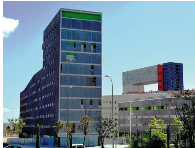
Fig. 15.7 Burgos and Garrido. 13 dwellings (EMVS) in the Sanchinarro PAU, Madrid, 2004–2007. Photograph of the outside, plan and sections
