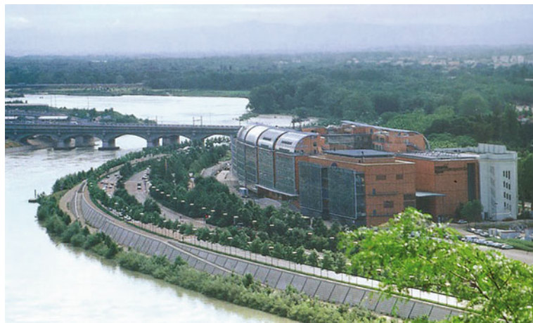
Fig. 25.7 Michel Corajoud and Renzo Piano, landscape project on the banks of the Rhône river and Cité Internationale. Lyon, 1991–2001
