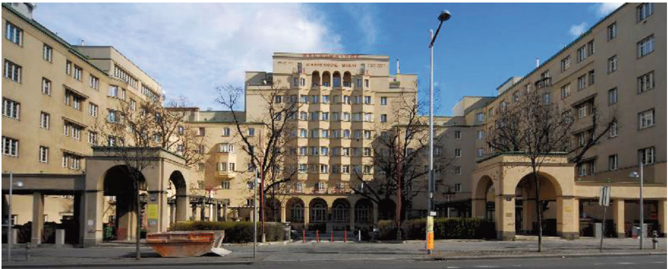
Fig. 3.8 Hubert Gessner, Reumannhof, Vienna, 1924–26, with 478 dwellings. View of the main entrance to the Hof
