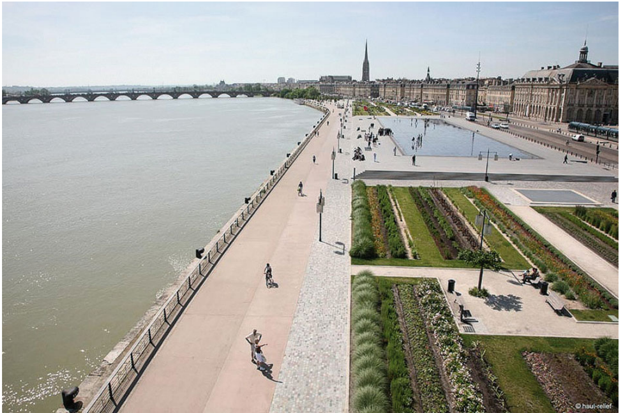
Fig. 13.6 Renovation of the riverside façade at “Place de la Bourse”, Bordeaux, 2009
