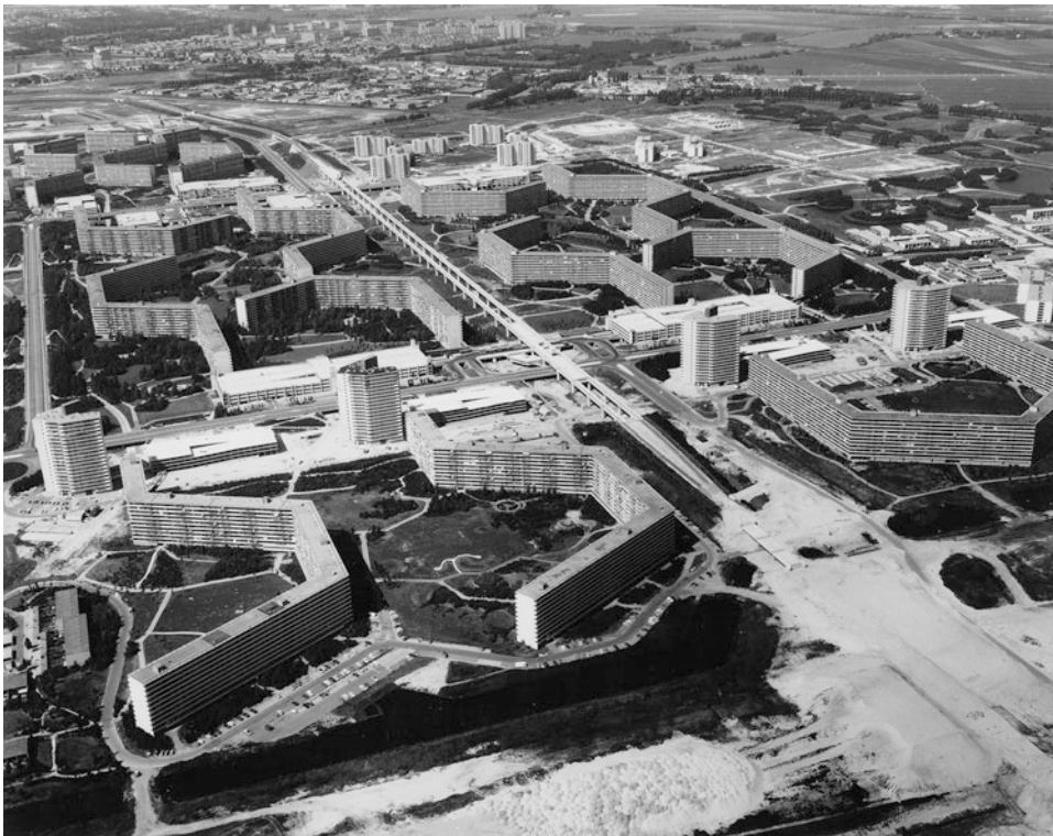
Fig. 7.2 Bijlmermeer, in Amsterdam, 1966–72, was presented as an advanced suburb in the motorised age, an achievement for the most radical functionalists. Nevertheless, this modernity soon became the icon of an acknowledged mistake. However, as is true in other cases, the urban and architectural designs were not the only factors to blame for the problems. In Holland, construction of Bijlmermeer coincided with the arrival of a large number of immigrants after independence of the former Dutch colony of Surinam in 1975
