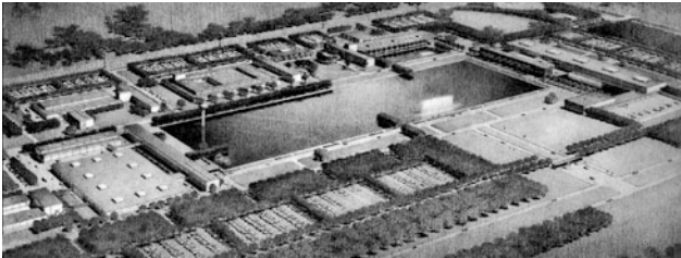
Fig. 19.7 Technical Centre of General Motors in Warren, Michigan, 1947–56. Project by Eero Saarinen
