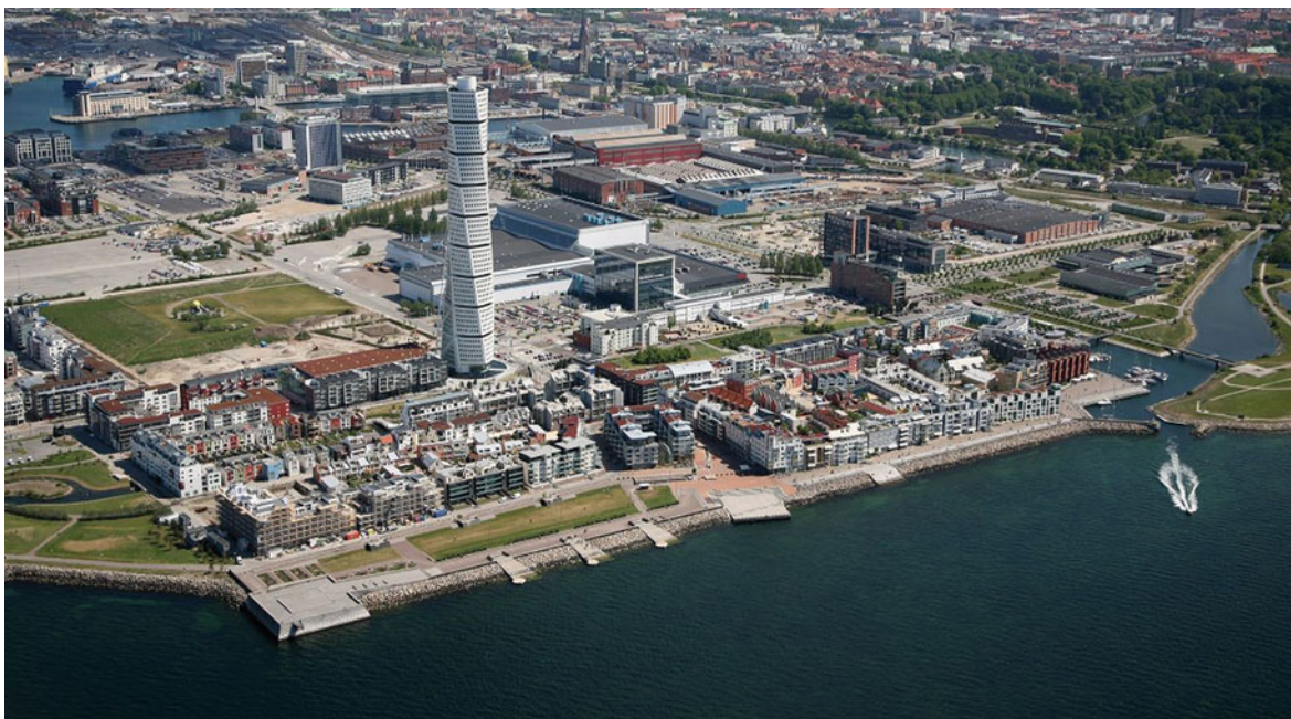
Fig. 21.4 Ecodistrict Bo01 in Malmö, Project by Klas Tham, 2001. Aerial view
