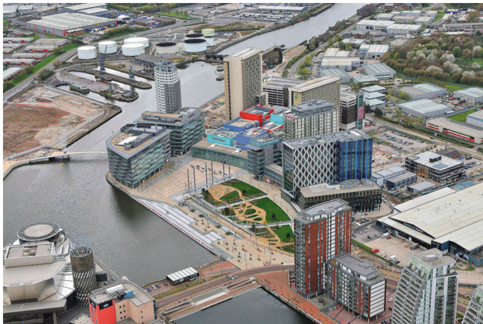
Fig. 21.8 Media city UK en Salford Quays, Manchester, UK, 2011. Aerial view
