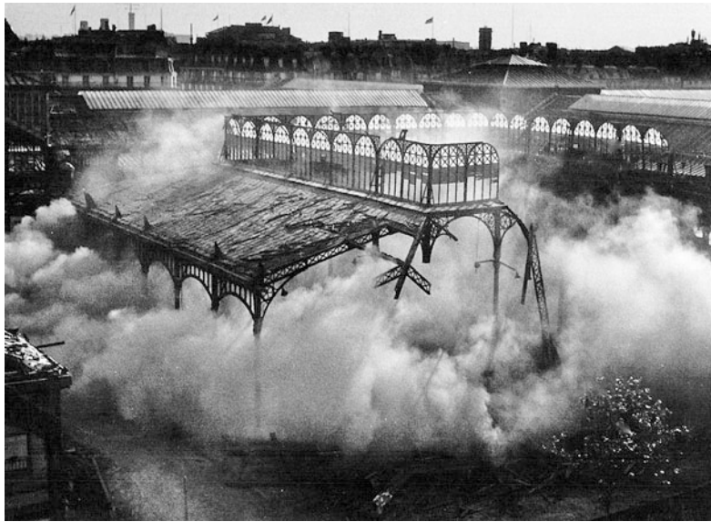
Fig. 12.1 Paris, the ‘Battle of Les Halles’: demolition of the market, 1972
