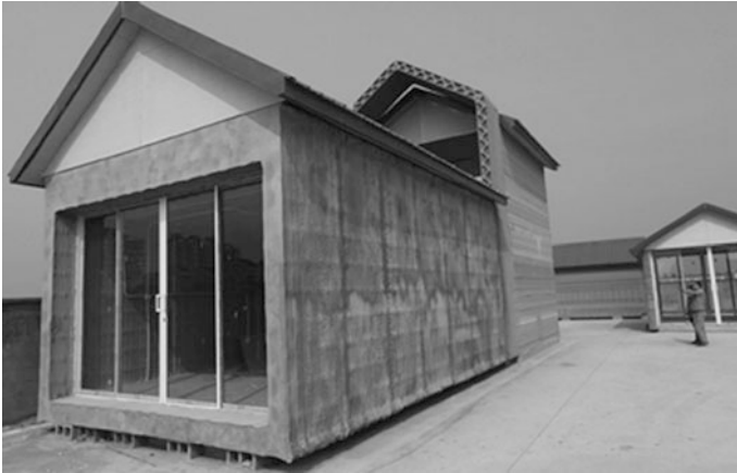
Fig. 6 One of the homes from the ANWAM 3D printed building project
