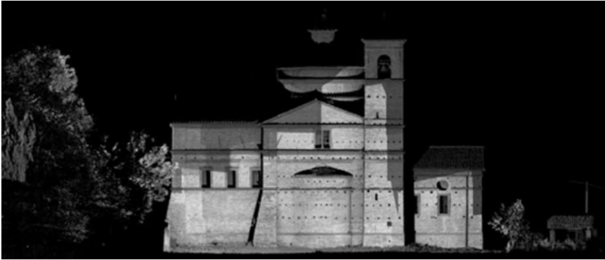
Fig. 2 Laser scanning of the church
