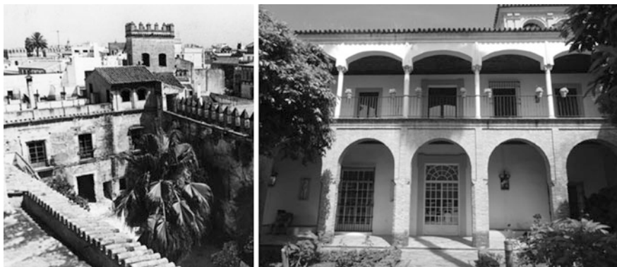
Fig. 5 Front of the Tennis Courtyard. Before and after the intervention
