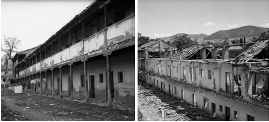
Fig. 7 The Casa de la Lona before and after its demolition. Photographs by Juan Antonio García Granados
