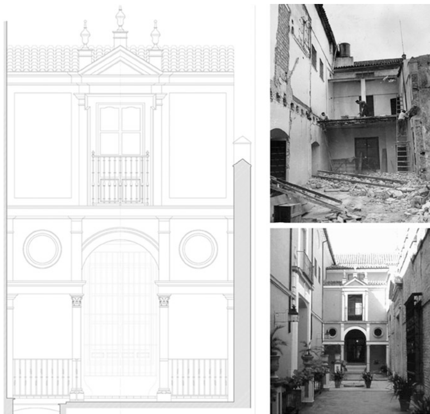
Fig. 7 Western façade of the courtyard at the north end of the Patio de Crucero before and after the intervention
