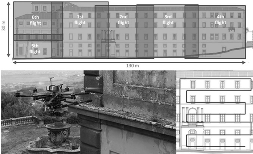
Fig. 5 Flight program (top), drone DJIA2 provided with GoPro Hero 3+ (on the bottom left), flight path (on the bottom right)
