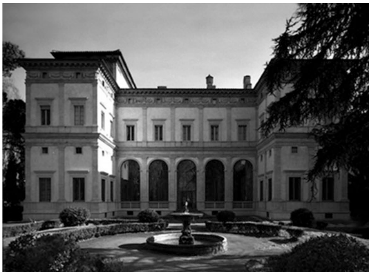
Fig. 1 Villa Farnesina, north façade
