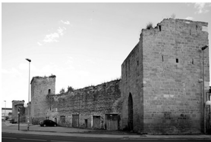
Fig. 1 View of one sector of the walls conserved
