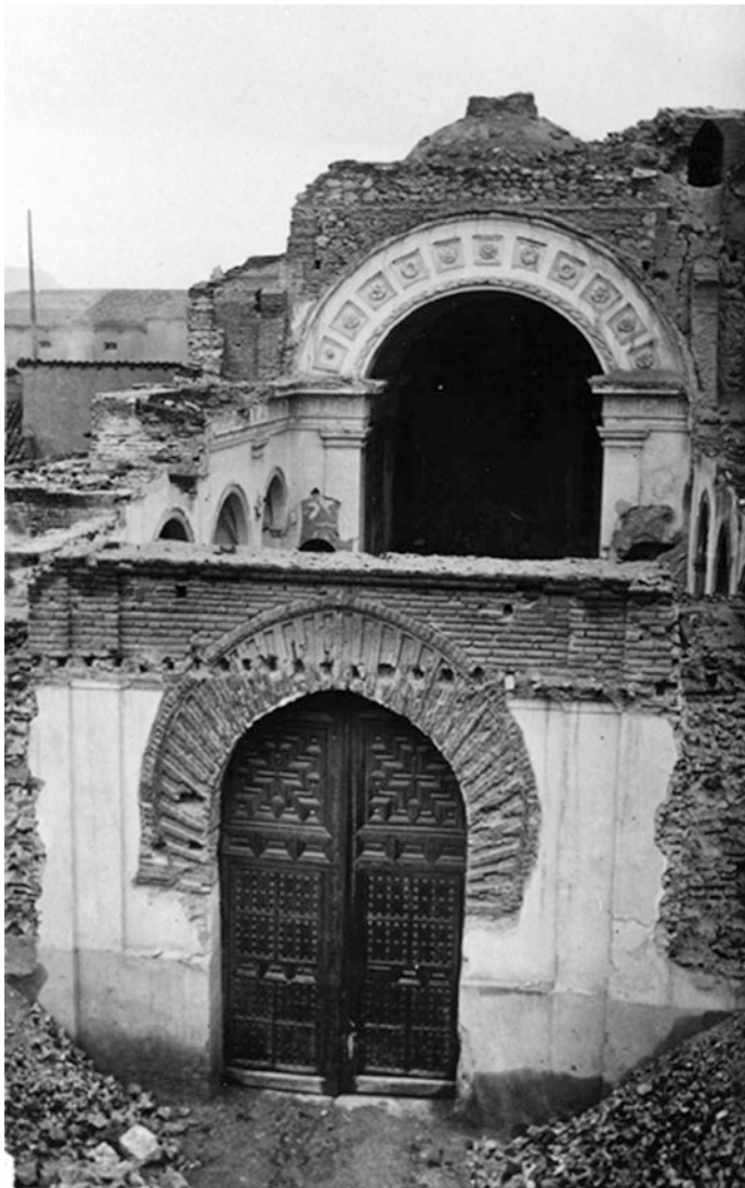
Fig. 6 Church of San Gil. Demolition process. Foto Goñi (AGA)
