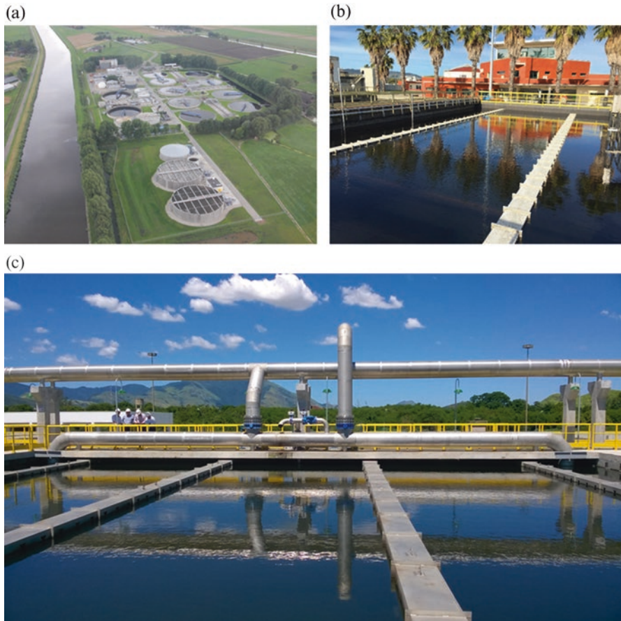
Fig. 4.11 Full-scale demonstrations of aerobic granular sludge technology. In (a), the granular reactors are displayed in the bottom of the picture (Provided by Royal Haskoning DHV). (a) Nereda® WWTP Garmerwolde, The Netherlands. Operation since 2013. (b) Nereda® WWTP Frielas, Portugal. Operation since 2014. (c) Nereda® WWTP Deodoro, Brazil. Operation since 2016
