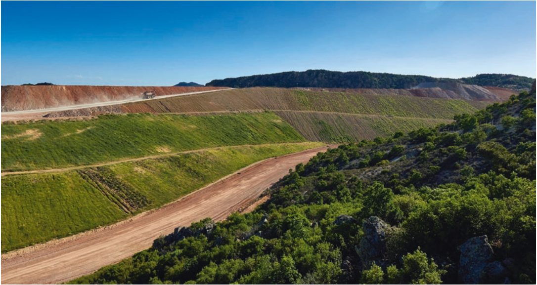
■ Fig. 7.24 Revegetated waste rock areas (Image courtesy of Eldorado Gold Corporation)
