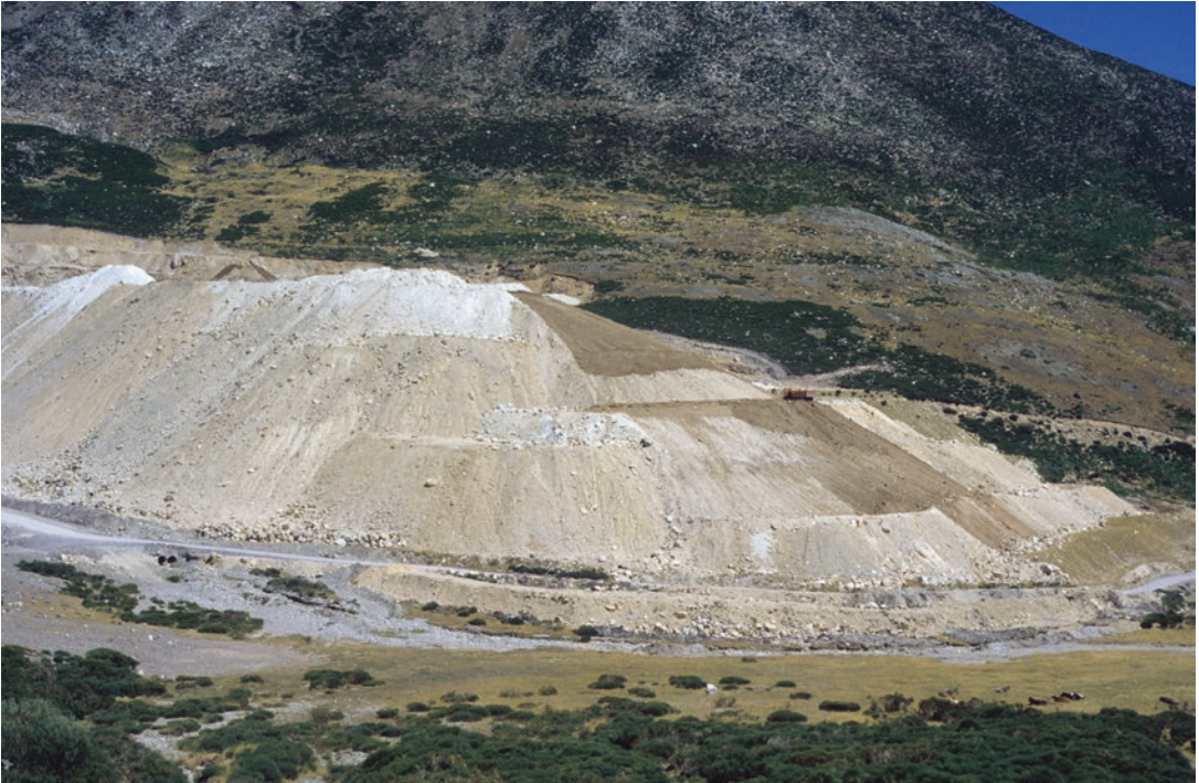
■ Fig. 7.1 Recontouring the waste dumps for reclamation (Spain)
