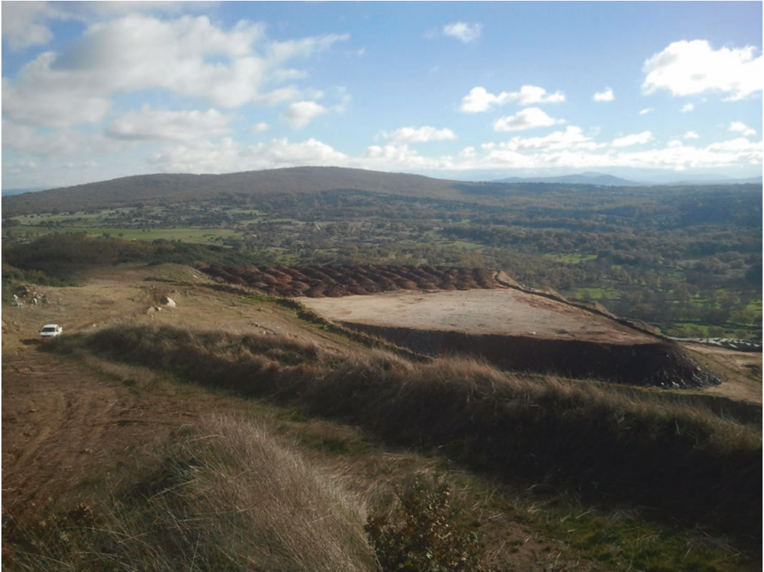
■ Fig. 7.12 Overburden (top soil) used for landscape contouring (Image courtesy of Daytal Resources Spain S.L.)
