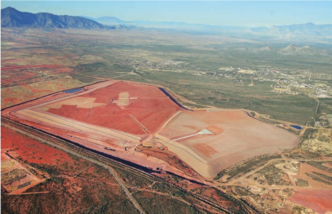
■ Fig. 7.48 Reclamation of North ( right ) and South ( left ) tailings impoundments as of 2013 (Image courtesy of FreePort-MacMoRan)
