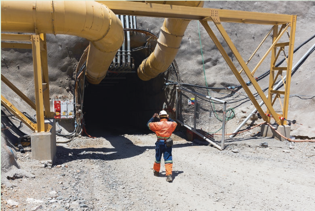
■ Fig. 5.41 Venetia decline to underground mine (Image courtesy of De Beers)
