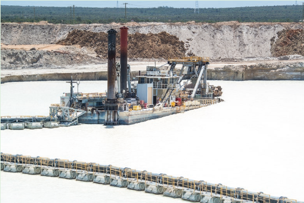
■ Fig. 5.38 Dredging operation (Image courtesy of Tronox)
