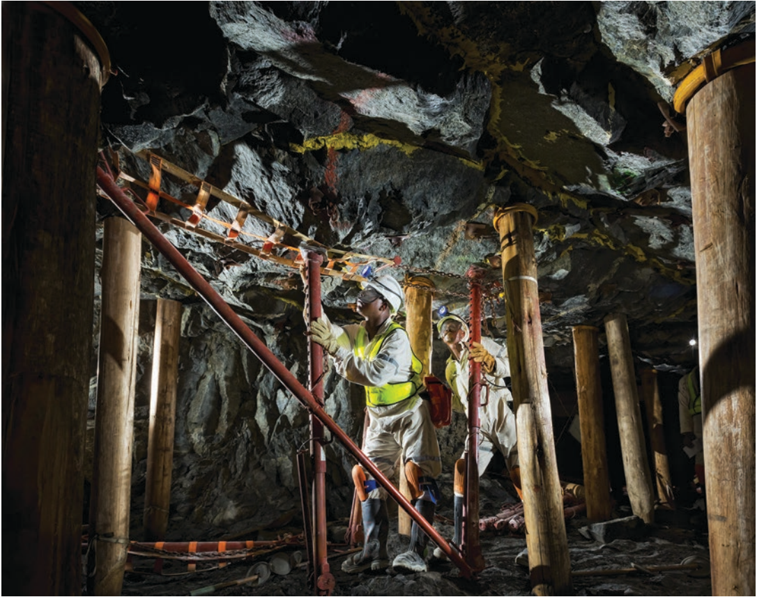
■ Fig. 5.57 Installation of canopy jack at Tumela Mine (South Africa) (Image courtesy of Anglo American plc)
