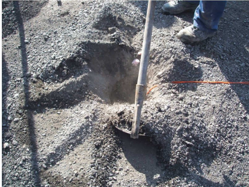
■ Fig. 5.89 Stemming of a borehole on top
