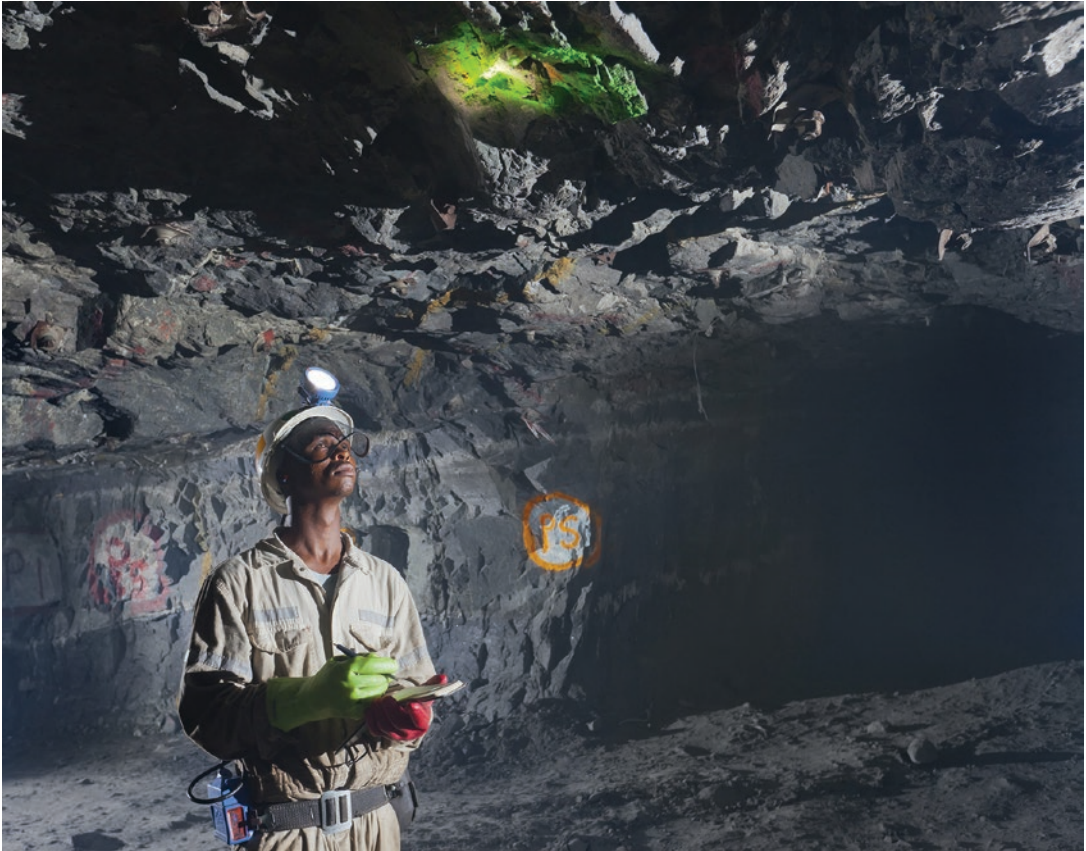
■ Fig. 5.47 Checking fall of ground (FOG) lights underground at central shaft in Bathopele platinum mine (South Africa) (Image courtesy of Anglo American plc)
