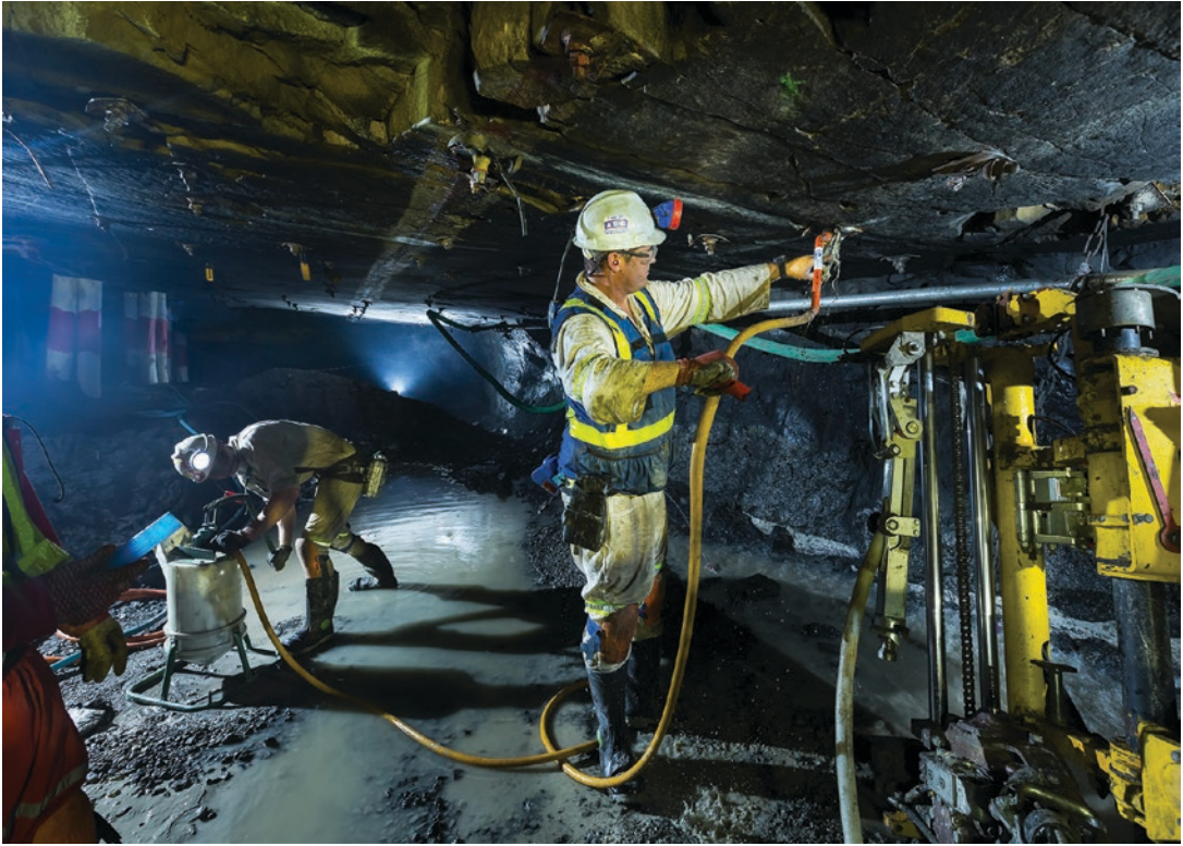
■ Fig. 5.54 Installing rockbolts at Bathopele mine (South Africa) (Image courtesy of Anglo American plc)
