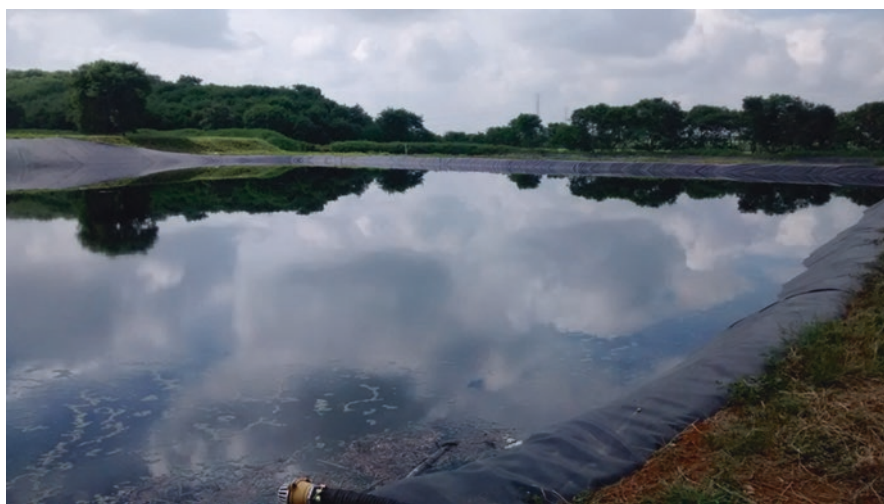
Fig. 5.10 Poned old leachate from the Navarro landfill (Source: Photographs by the authors 2013)
