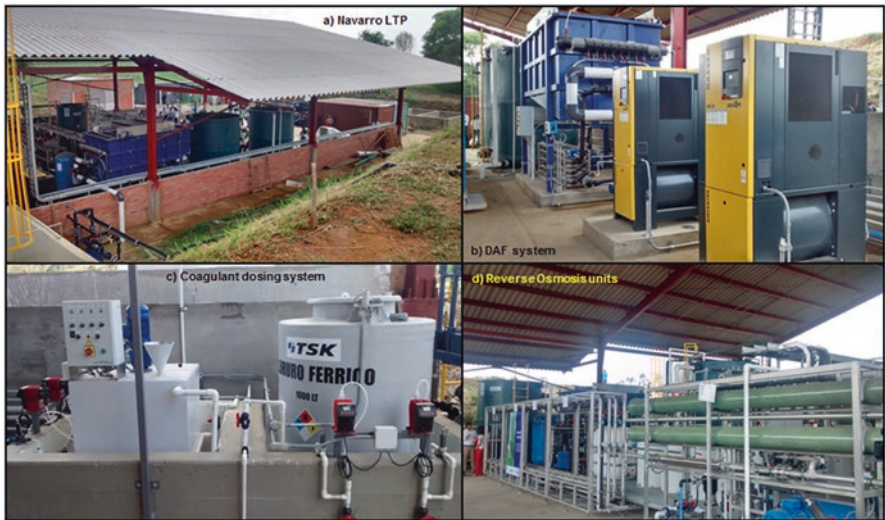
Fig. 5.12 Photographs of the Navarro landfill leachate treatment plant (Source: Photographs by the authors 2014)
