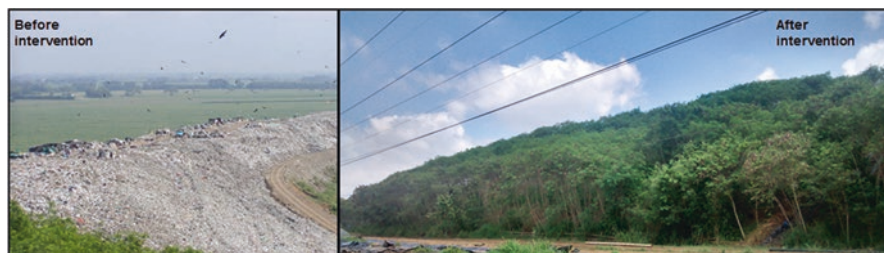
Fig. 5.9 Navarro landfill – before and after intervention (Santiago de Cali, Colombia) (Source: Pueblo 2012, Photographs by the authors 2014)
