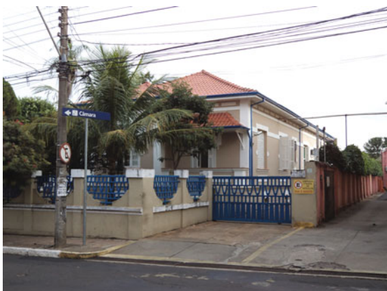
Fig. 13.4 Superintendent's House, 2012. Source: Authors' collection (2012)
