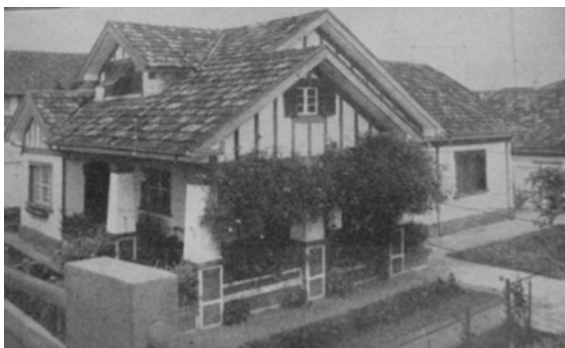
Fig. 13.8 Residence no. 35 na Vila Noroeste, 1960. Source: Revista NOB (no 290, 1960)
