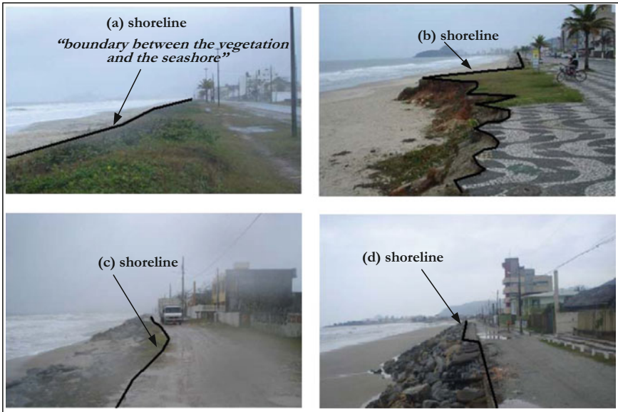
Fig. 15.1 Examples of definition of a shoreline; a the shoreline is the boundary between the vegetation and the seashore while in b, c, d , the shoreline is the boundary between the continent and the portion adjacent to the sea where there is no effective marine action beyond the maximum reach of the waves, characterized by urban settlement and problems of coastal erosion. Source Gonçalves [18]
