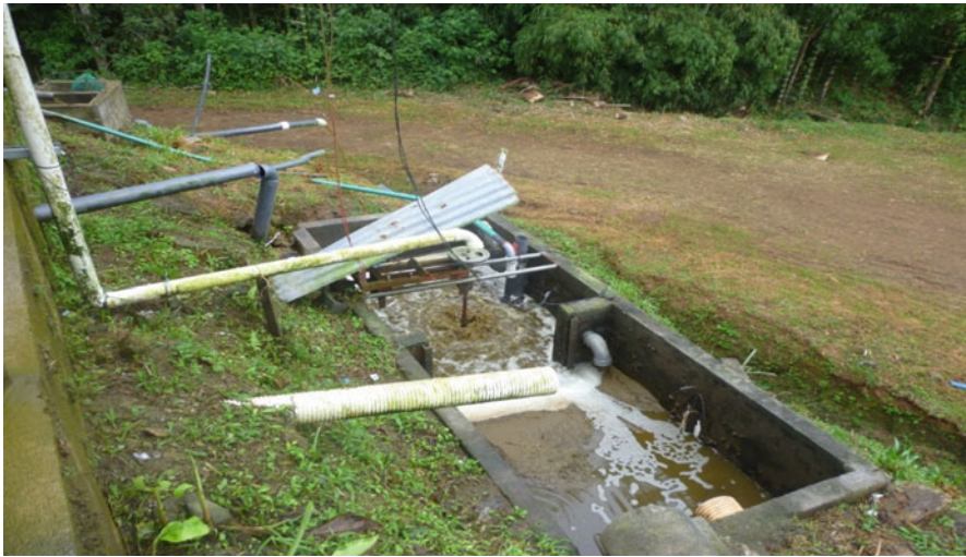
Fig. 4 Separator tan of purines and biomass and the pump system
