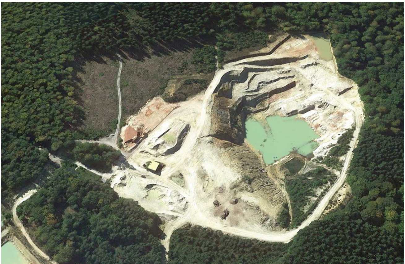
Fig. 5.4 The Transinne quarry cuts into Lochkovian shales and sandstones outcropping on the Selandian erosion surface of western and central Ardenne, here at 445 m asl, exposing a \sim 65 -m-thick mantle of deeply kaolinized rocks (© Google Earth 2015)
