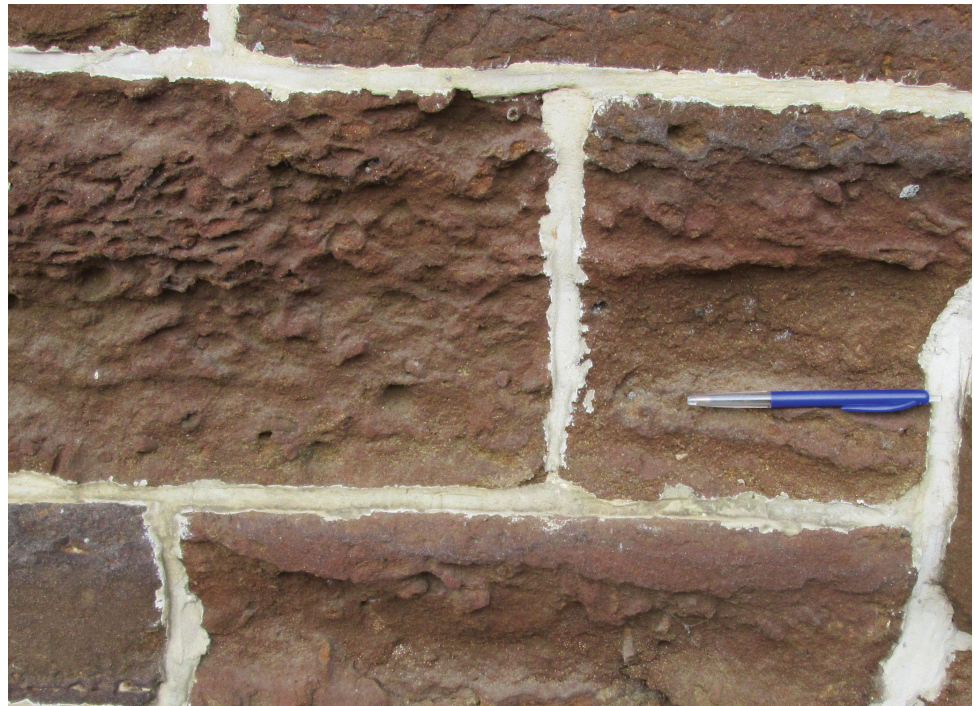
Fig. 14.12 Zoom on the stone front of the Testelt water mill, built in 1608. Note wear of the building blocks of local ironstone extracted from the Diest Formation
