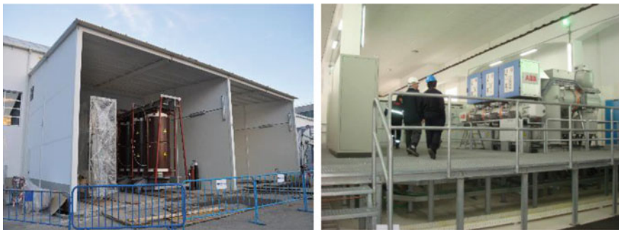
Fig. 2 Installation of HiDry 72 (12 MVA) in the bay ( left ). GIS installation ( right )
