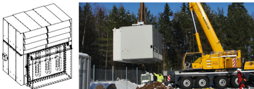
Fig. 4 Enclosure for outdoors ( left ). Unloading of HiDry 72 (16 MVA) with the enclosure ( right )
