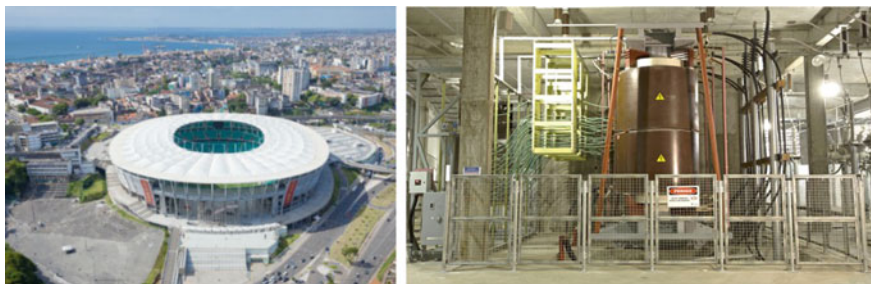
Fig. 3 Fontenova stadium overall view ( left ). HiDry 72 (25 MVA) and OLTC installation ( right )
