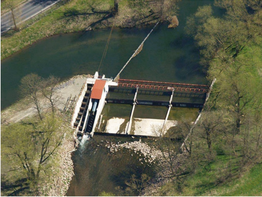
Figure 9 Screw supplied by residual flow from the Werra River near Meinigen, Germany
