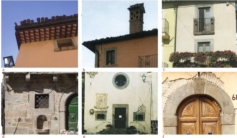
Fig. 4. Examples of Retrosi building elements: (a) roof with decorated rafter tails; (b) brick chimney; (c) (d) (e) portals and windows in grey sandstone or limestone; (f) keystone decorations with medieval iconography.
