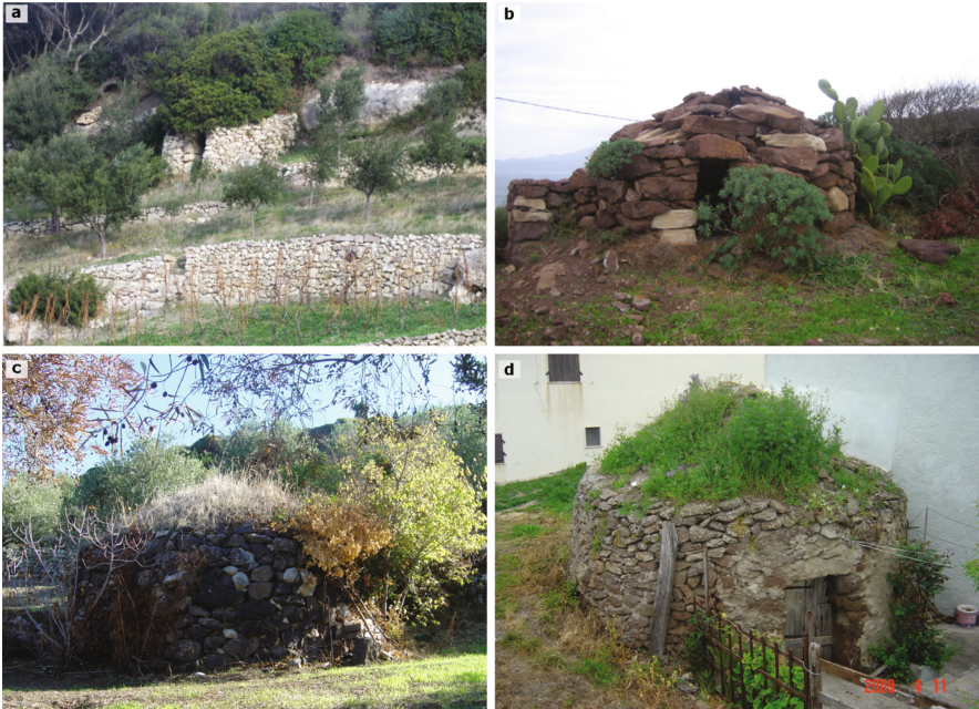
Fig. 3. Different materials used in some locality within the coastal Planargia of Bosa; (a) Badde Uraghe/San Nicola (Magomadas); (b) Santa Maria del Mare (Magomadas); (c) Lampis (in the north slopes of Magomadas); (d) Chele, in the seaside of Magomadas. The materials are the late Miocene sedimentary lithologies or ignimbrites of the cast-alkaline cycle oligo-Miocenic or the Pliocene basalts [7, 8].
