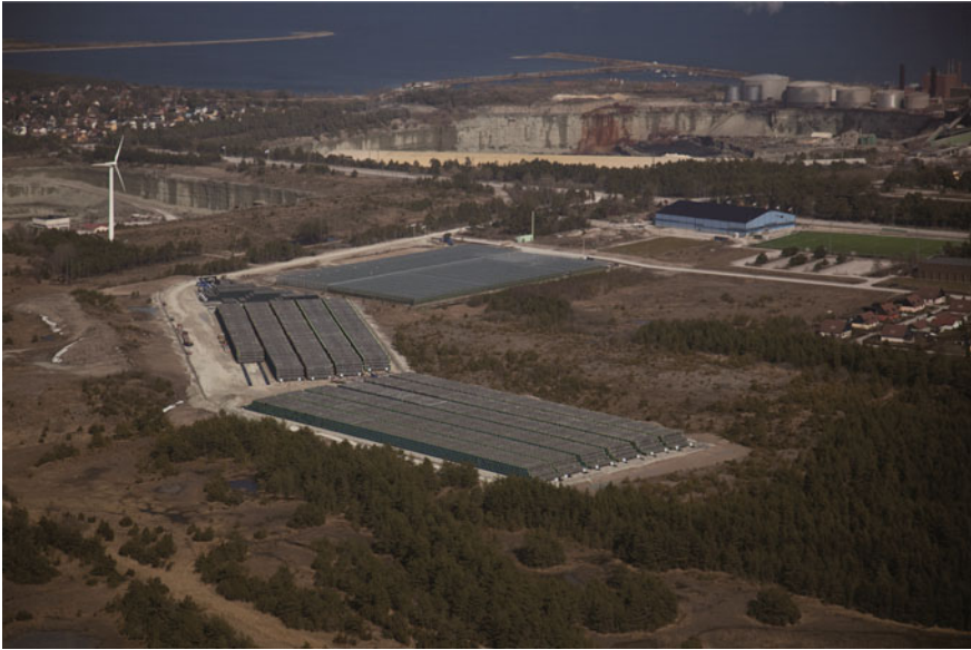
Fig. 8.5 Nord stream pipeline Marshalling Yard, Slite, Sweden ( source Nord Stream AG)
