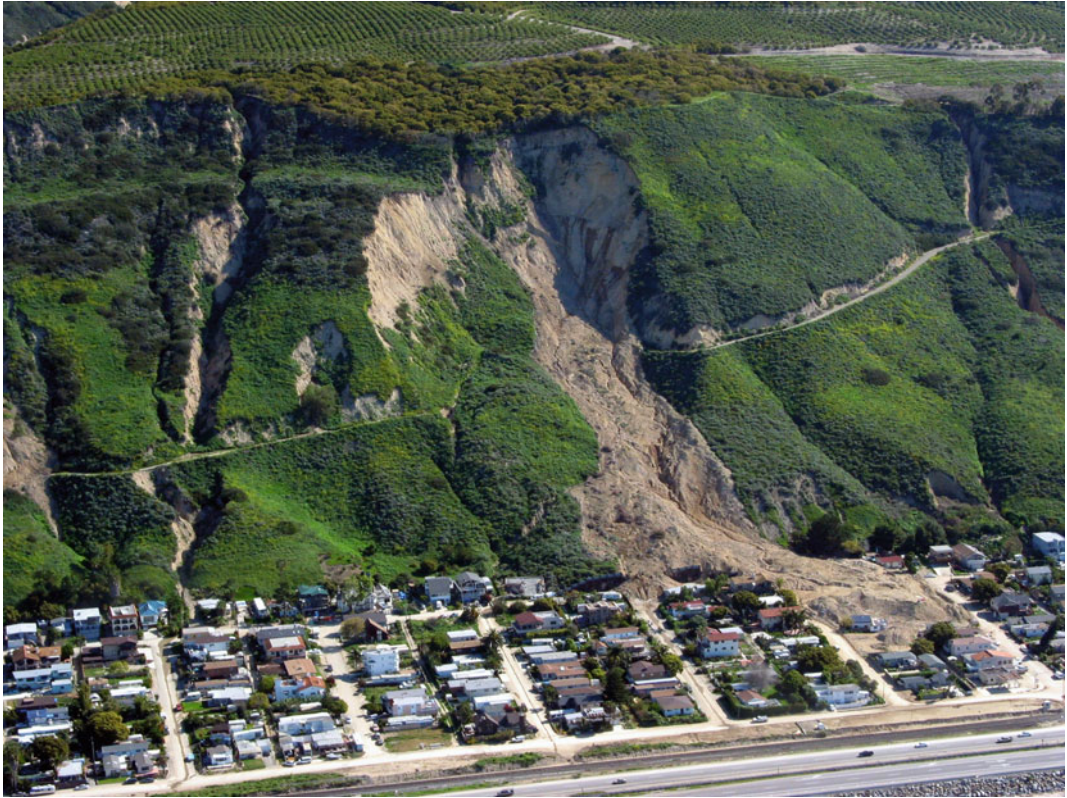
Fig. 35 The 1995 La Conchita, California (USA) earthflow occurred after heavy rains. No one was killed or injured, as it moved relatively slowly. This landslide later reactivated in 2005, and moving much more rapidly, killed 10 people. Photo by Mark Reid, U.S. Geological Survey
