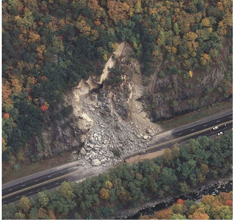
Fig. 3 This rockfall in North Carolina (USA), occurred on a highway through Pigeon River Gorge, on October, 2009, and caused traffic delays for weeks. Photo by North Carolina Department of Transportation
