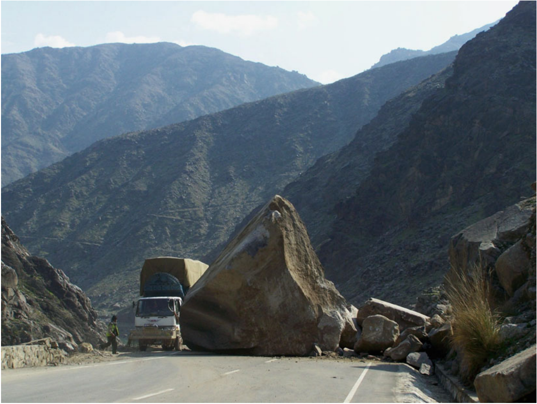
Fig. 5 Jalalabad Road, Afghanistan—Rockfall on the Jalalabad Road which is a highway from Kabul to Surobi and Jalalabad, Afghanistan, February 28, 2007. Photo by
