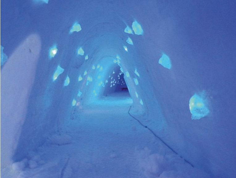
Fig. 28.2 Arch snow tunnel (Photograph: Kai Rynnänen 2011)
