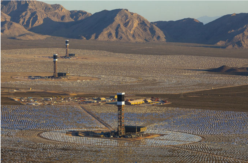
Fig. 12 An aerial view of the 392 MW Ivanpah concentrated solar power tower facility at sunrise, showing three towers. Picture taken from US DOE website with permission [40]
