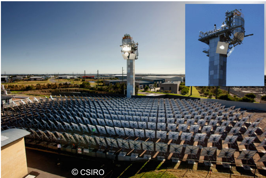
Fig. 11 1.2 MW Concentrated Solar Power research and demonstration facility at CSIRO Energy Centre, Newcastle, Australia [39]
