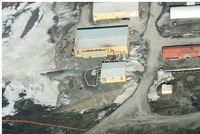
Fig. 28.3 Standby Power Plant Spill of 2007. The area outlined in white indicates the extent of the soil excavated (aerial photo Google Earth)
