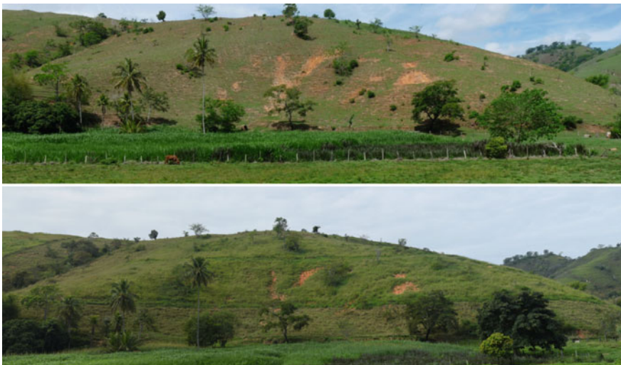
Fig. 5.2 Illustration of slope of pilot area at Itaocara, Rio de Janeiro from 06/2015 ( above ) and 06/2016 ( below ), © Roman Seliger
