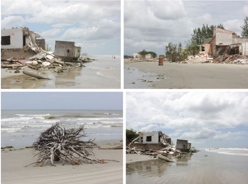
Fig. 24.2 Houses destroyed by coastal erosion in Ponta Norte of Ilha Comprida (2013)
