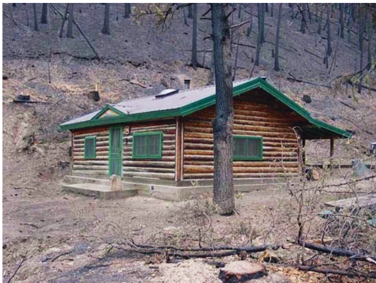
Fig. 11.5 The Bar Gulch Cabin (Helena National Forest) survived a wildfire in 2000, because it was protected by fire retardant wrap and a water sprinkler system. Historic structures will be vulnerable if fire frequency increases in the future (Photo by Carl Davis, U.S. Forest Service)
