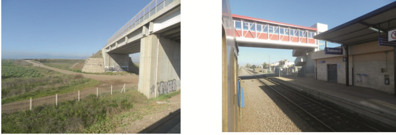
Fig. 12. General obstacles in Sardinia pilot site [12]
