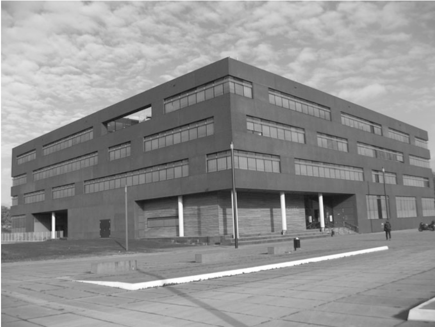
Fig. 6.3 The CITEC building on the Bielefeld Campus with automatic blinds for sun protection lowered. Source Ulrich Schramm
