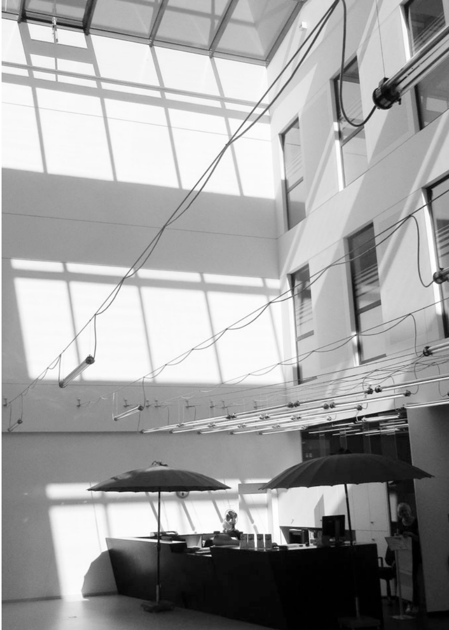
Fig. 6.6 Atrium in the library with improvised sunshades for the librarians. Source Ulrich Schramm
