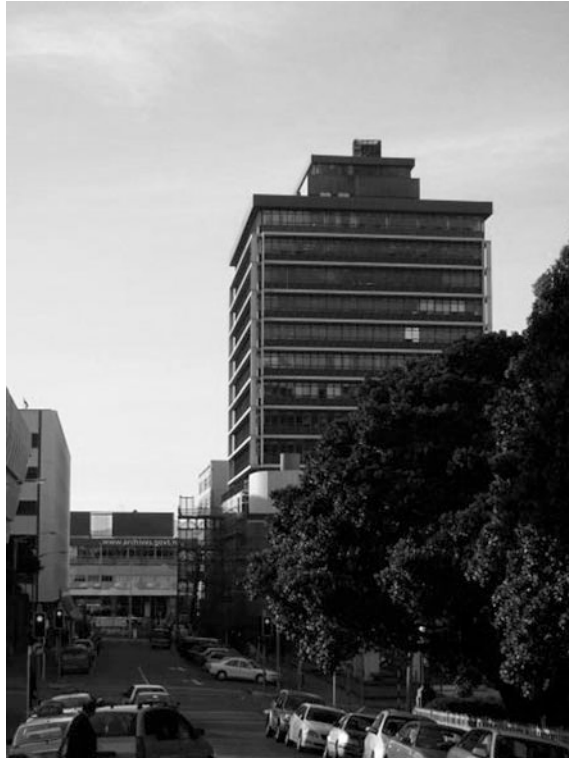
Fig. 13.1 MWD Head Office Building in Wellington. Source Author
