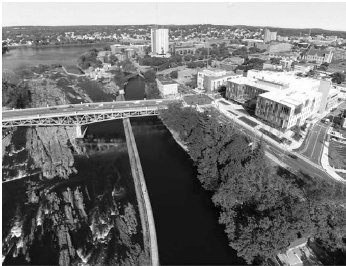
Fig. 21.1 University Crossing, UMass Lowell: Student center with ground level retail along the campus edge. Source Edward Dudley, Perkins + Will
