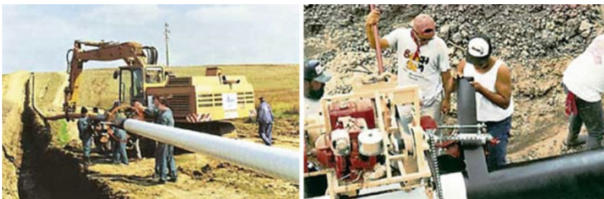
Fig. 9 Rehabilitation of the damaged pipe section using cold-pack band
