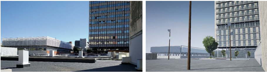
Fig. 1. Picture of the actual building next to the barcelona school of architecture (left) and virtual environment with the renovation proposal (right).
