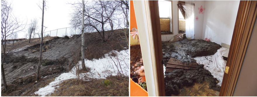
Fig. 37.2 Example of the consequences of a shallow landslide. The debris slammed into the house located at the toe of the slope
