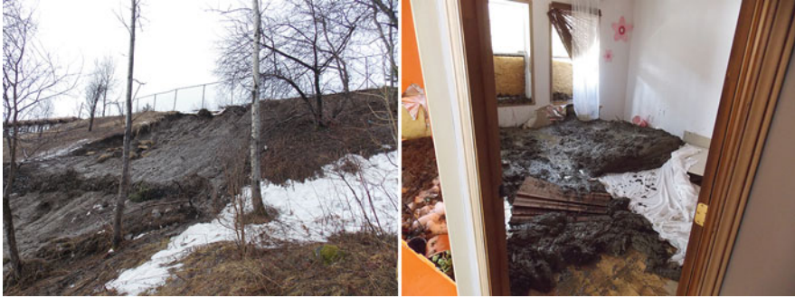
Fig. 37.2 Example of the consequences of a shallow landslide. The debris slammed into the house located at the toe of the slope
