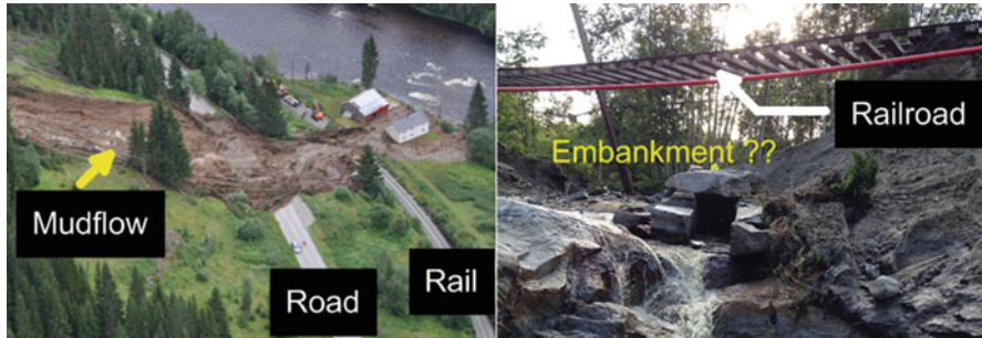
Fig. 46.3 Examples of the impact of extreme weather on the Norwegian transportation infrastructure (Source: NNRA and NPRA)
