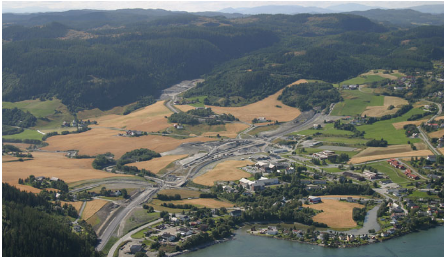
Fig. 43.1 Construction work in areas of marine clay in Norway is challenging, and requires large amounts of ground investigations. The picture is from building of the new E39 in Børsa, Mid Norway (Photo: NVE 2004)
