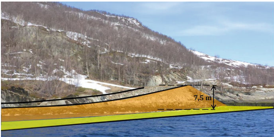
Fig. 35.8 Reconstruction of the embankment fill for the road along the shoreline of Sokkelvik prior to the landslide in 1959 (Modified from Austefjord 2015)
