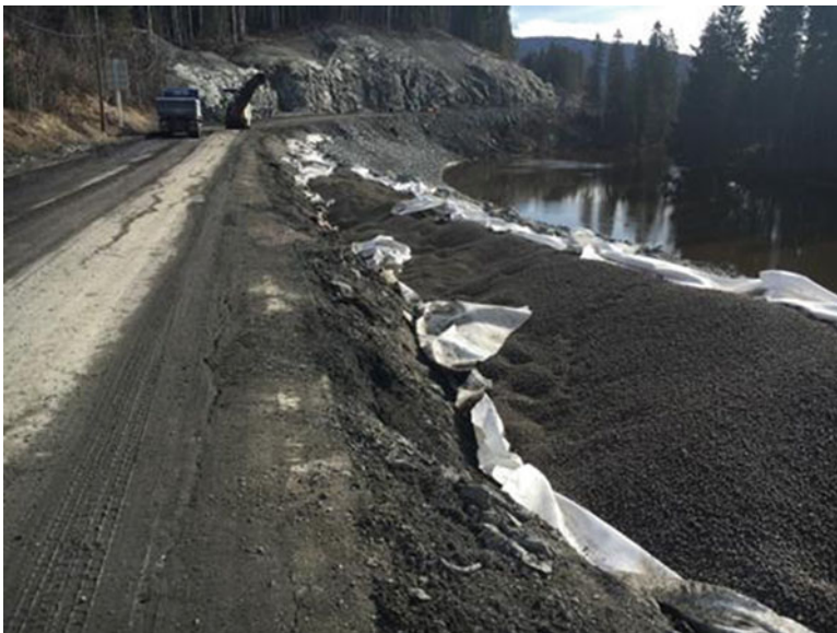
Fig. 33.4 Filling with lightweight material (Photo: T. Flobak, Rambøll)
