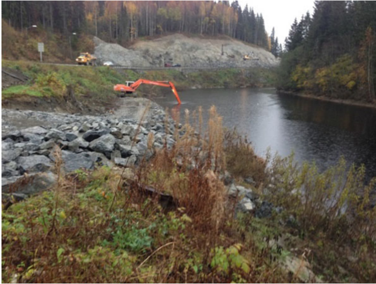
Fig. 33.5 Building of erosion protection (Photo: T. Flobak, Rambøll)
