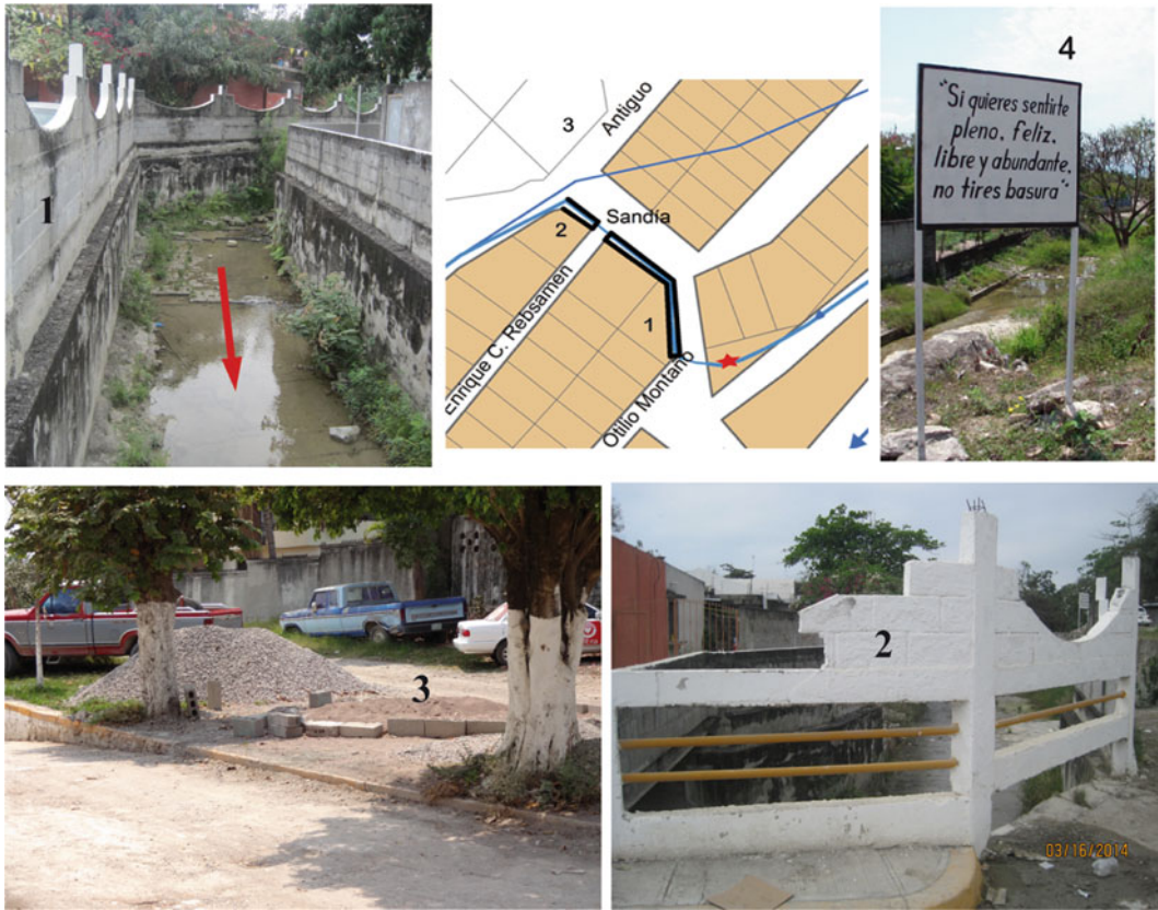
Fig. 4 Adjustments made by the Magisterial neighborhood committee. The map indicates its location. The star shows the streambed curve modified to create a backwater. (1) Retaining wall of the stream (black line in the map). (2) Modifications in the retaining wall to enhance
