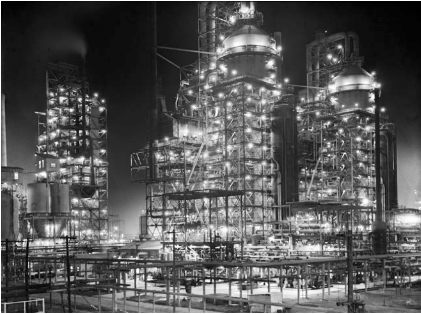
Fig. 1 Catalytic Cracking Units, Standard Oil of New Jersey Baytown Refinery, 1946. Credit Standard Oil of New Jersey Collection, Image Number 43680, Archives and Special Collections, University of Louisville.
