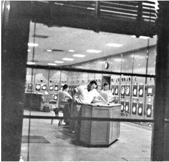
Fig. 3 Cat Cracker Control Room, Shell Oil Deer Park Refinery. Credit United Steelworkers Local 13-1, Pasadena, Texas.
