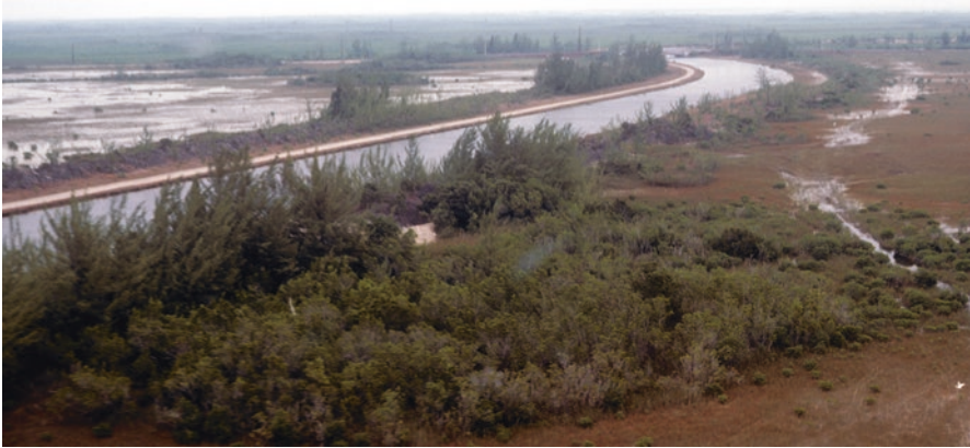
Fig. 1.9 Example of a drainage canal in the southeastern portion of the Florida Everglades that is also used for boat (barge) traffic. The C-111 Spreader Canal Western Project was designed to provide ecosystem restoration of freshwater wetlands, tidal wetlands, and near-shore habitat in addition to flood protection maintenance and recreation opportunities. Located in south Miami-Dade County, the project includes pump stations, detention areas, culverts, conveyance canals, and 10 plugs/water control structures. Note the presence of an elevated gravel service road ( left side of photo) parallel the canal and airboat trails ( right side of photo) on the other side. Exotic invasive species (e.g., Casuarina ) have colonized the canal margins. Casuarina is a genus of 17 tree species in the family Casuarinaceae, native to Australia, the Indian Subcontinent, southeast Asia, and islands of the western Pacific Ocean. These evergreen shrubs and trees grow to 35 m tall. The foliage is slender, much-branched green to grey-green twigs bearing minute scale-leaves in whorls of 5–20. The flowers, simple spikes, are produced in small catkin-like inflorescences. Most species are dioecious, but a few are monoecious (Credit: C.W. Finkl)
