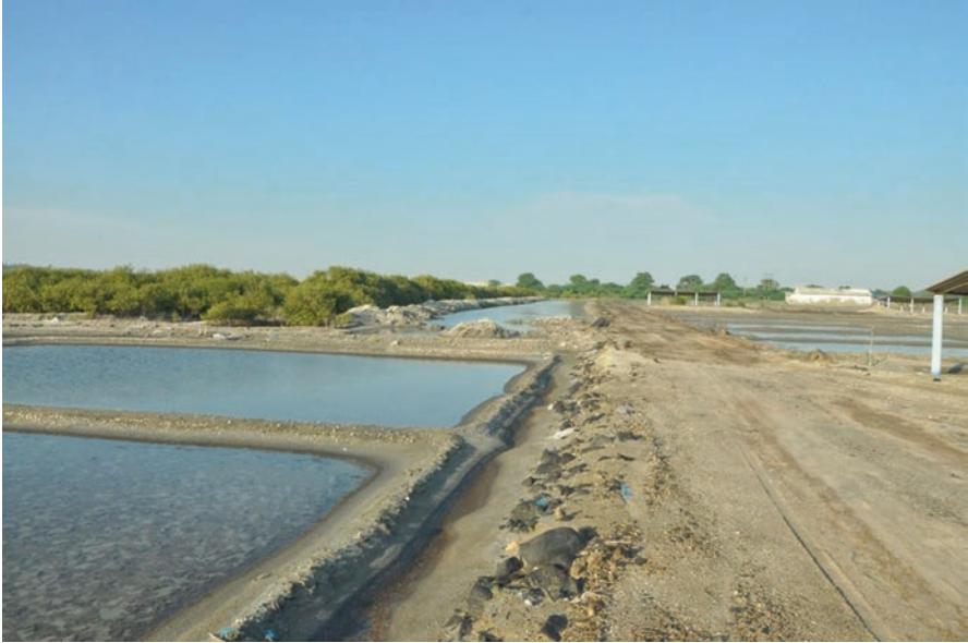
Fig. 12.3a Newly constructed salt pans
