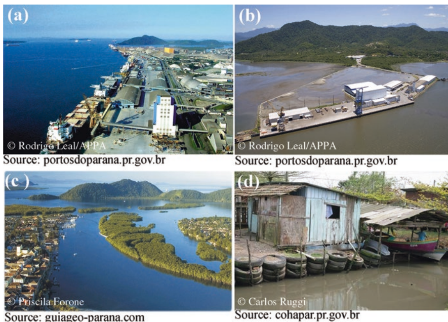
Fig. 16.16 Anthropogenic impacts affecting the Paranaguá Estuary. (a) Paranaguá port, a maritime terminal for grain and other agro-industrial products; (b) Pontal do Felix port, a recently port facility with intense dredging activities; (c) urban settlements (Paranaguá city); (d) direct sewage discharge in the upper reach of the estuary related to riverside communities
