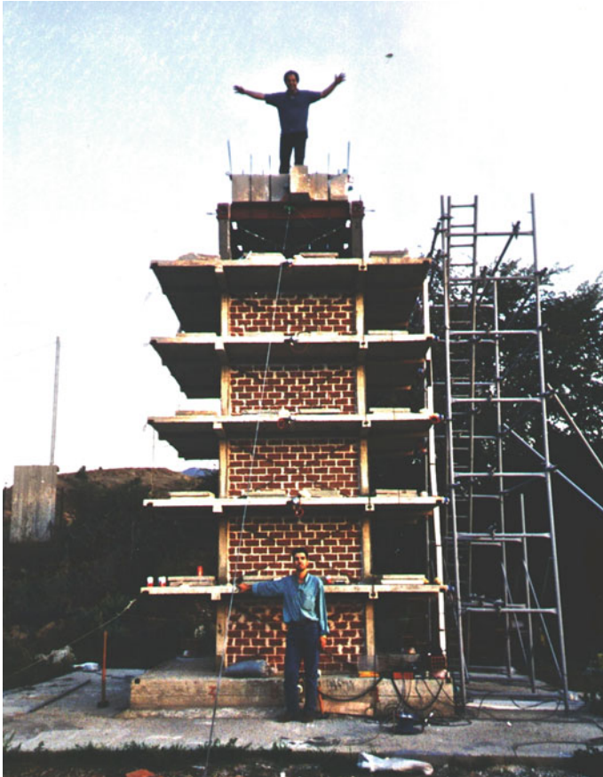
Fig. 4.3 The 6-story model structure (Masonry scheme 2b, September 1997–January 2004)
