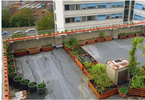
Fig. 14.5 Rooftop garden in Bologna (Credit: Orsini)
