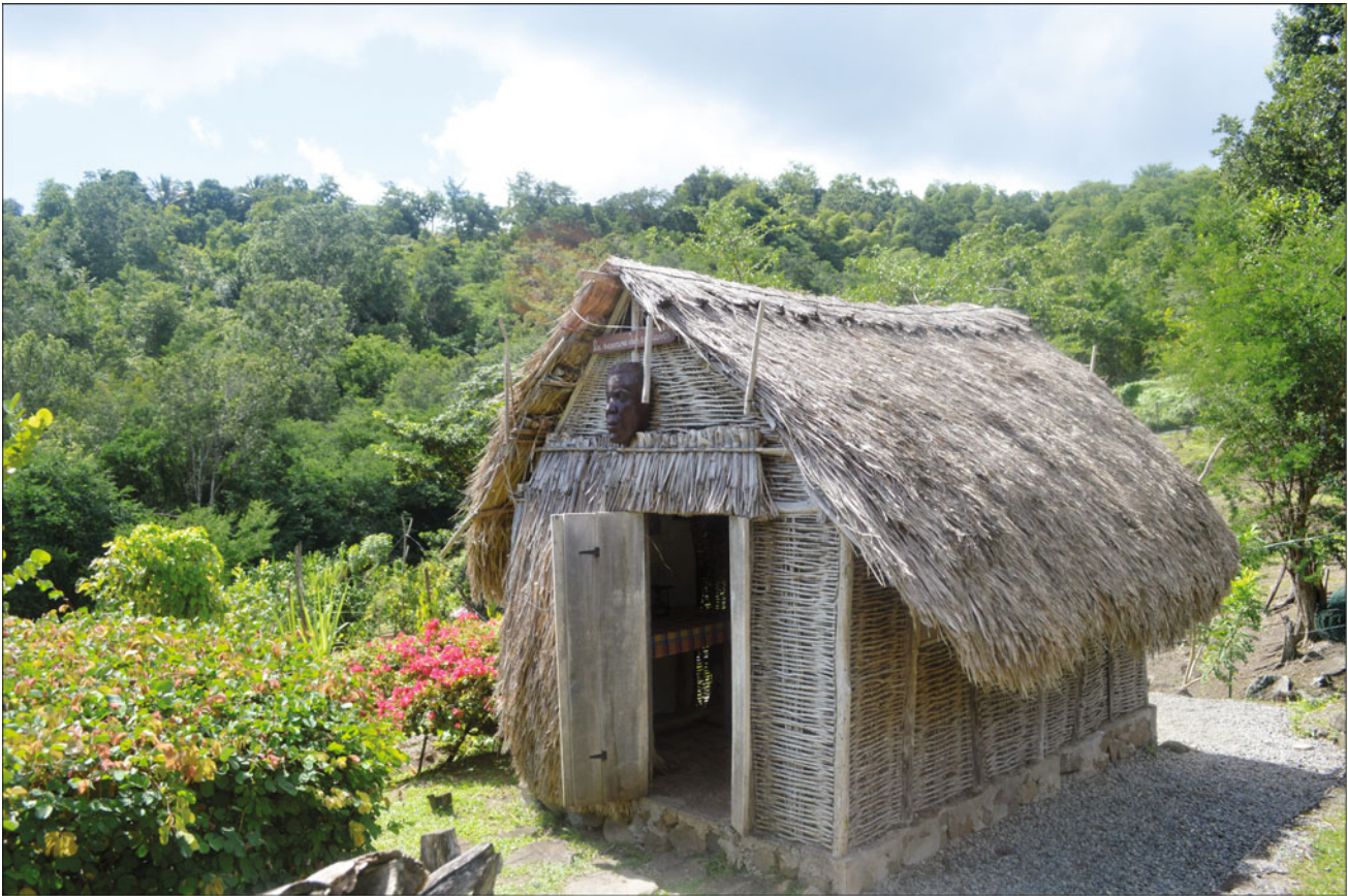
Fig. 12.7 Two-room cabin built in the style and with the materials often used by rural Black Martinicans both before and after emancipation. While this structure is not representative of all of the housing types occupied by formerly enslaved people, it does demonstrate a
