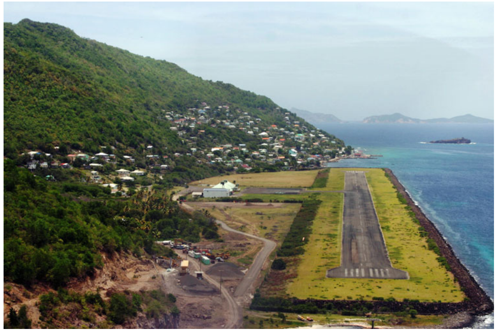
Fig. 15.7 Aerial view of the J.F. Mitchell Airport on the southern coast of Bequia. Photograph by A. Ollivierre
