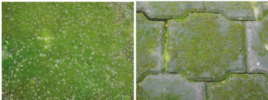
Fig. 1.3 If the conditions are right, lichen will consume and grow on the concrete as on any other soil
