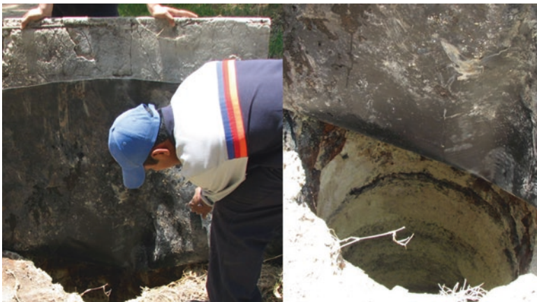
Fig. 2.3 Sulfur deposits at the visiting manholes of experimental site
