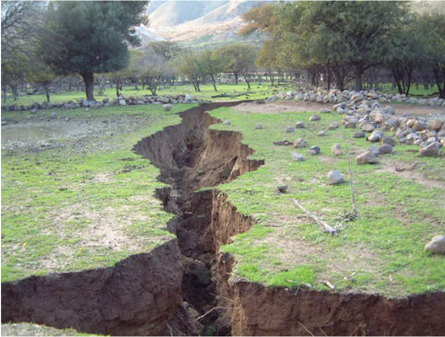
Fig. 3.14 Surficial, up to 10 m deep ruptures in the central part of the Lakki plain, which formed during the first episode in November 2001. Neither vertical nor
