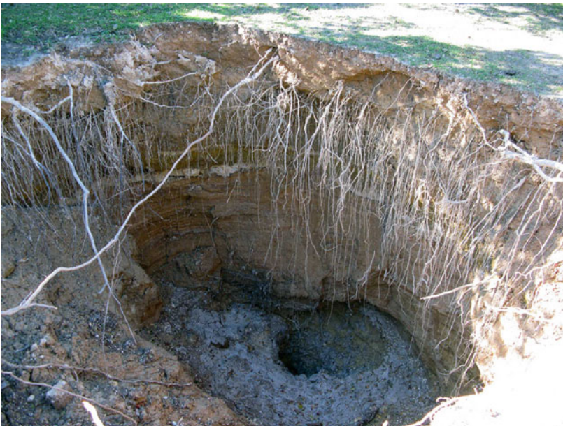
Fig. 3.17 6–8 m deep and 8 m in diameter “doline-type” hole next to the rupture of November 2011. The filling was washed away through a drainage
