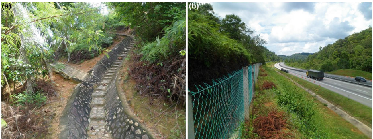
Fig. 4.9 Field verifications of detected landslide
