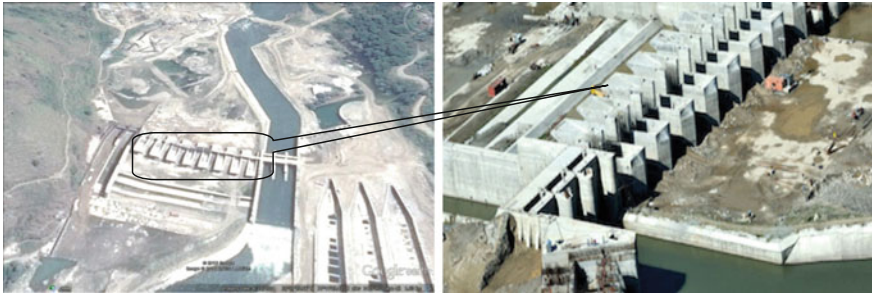
Fig. 2 Google map of PKW (Sawra Kuddu HEP) and on site map of PKW (Sawra Kuddu HEP) (Ref HPPCL)
