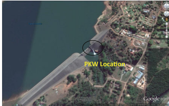
Fig. 4 Spatial location of Tzaneen Dam PKW (Ref Google Earth)
