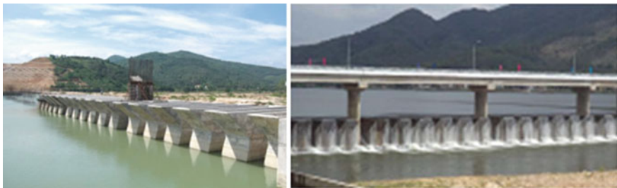
Fig. 6 Under construction and constructed PKW at Van Phong Dam (Vietnam)
