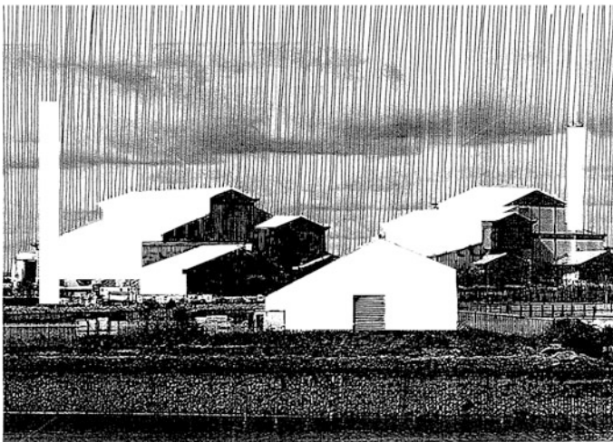
Fig. 7 Federico Segat, Ash Lines , 2016. Teesside WTE Power Station, Billingham
