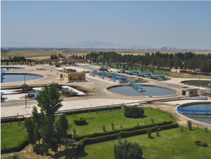
Fig. 8.1 View from the digesters of WWTP Isfahan North
