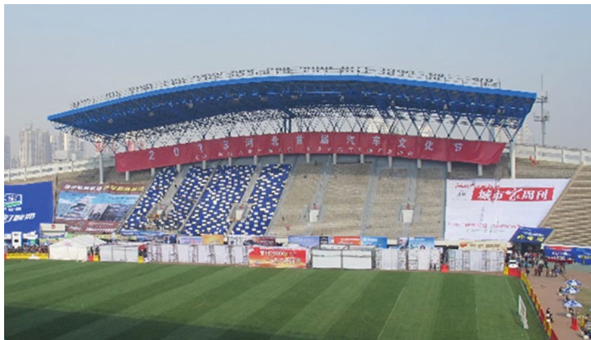
Fig. 17.8 The space truss of the stadium
