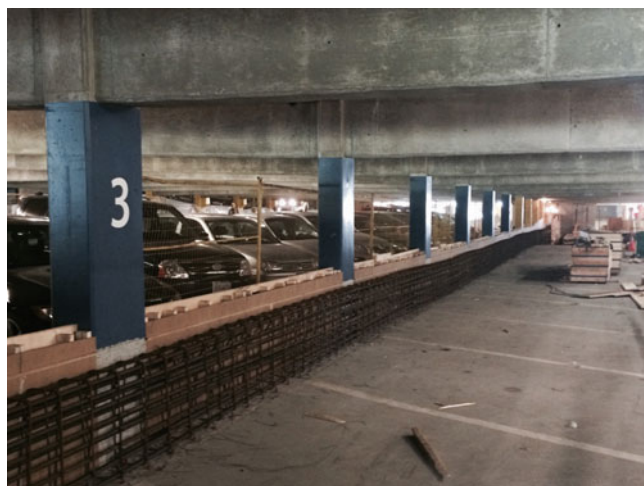
Fig. 16.7 New reinforced concrete beam, under construction
