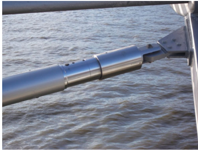
Fig. 2.5 Moving end of pier damper over the River Thames
