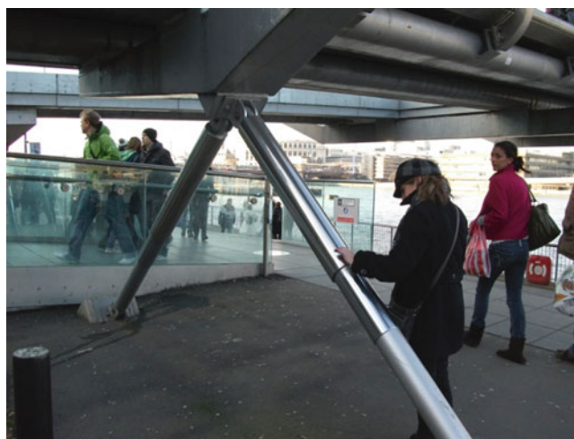
Fig. 2.9 Vertical damper pair with pedestrian access
