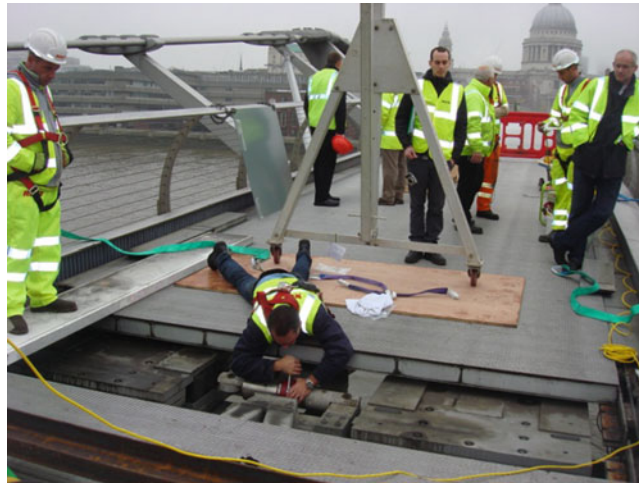
Fig. 2.7 Deck panels removed deck damper showing
