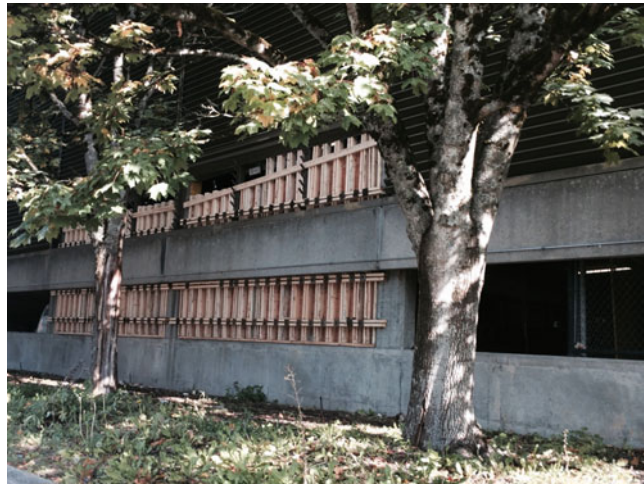
Fig. 16.5 New external shear walls, during construction
