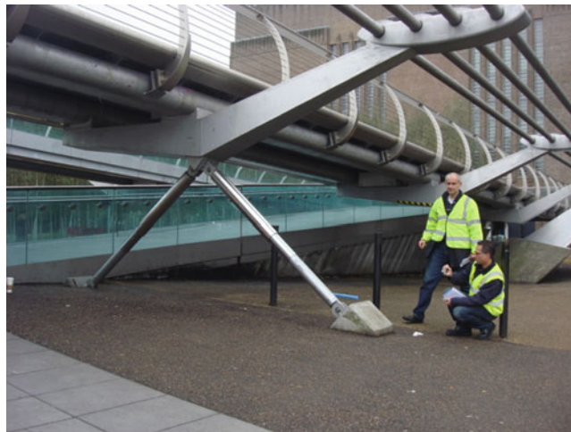
Fig. 2.7 Deck panels removed deck damper showing
