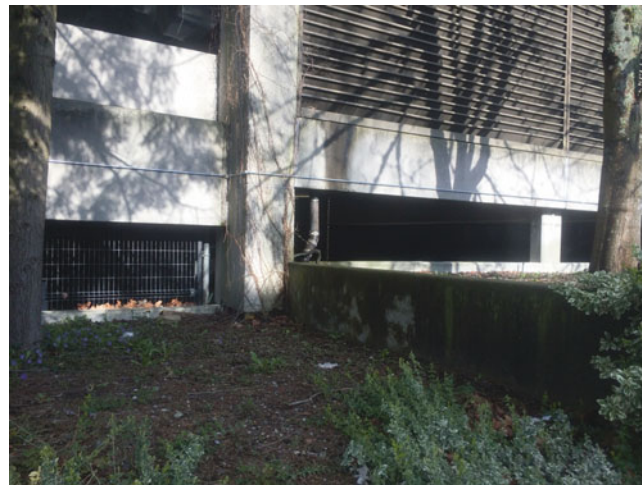
Fig. 16.4 External shear wall and short columns, before upgrade
