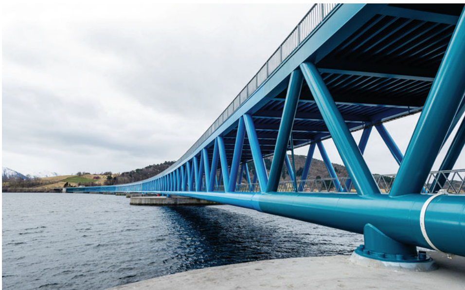
Fig. 14.1 The Bergsøysund Bridge. Photograph by NTNU/K. A. Kvåle
