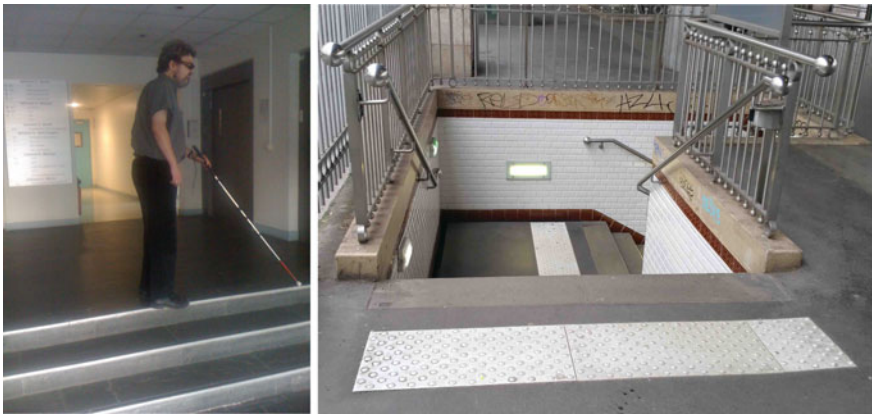
Fig. 5 Using a white cane ( left ) and a tactile warning surface ( right ) to identify the top of stairways
