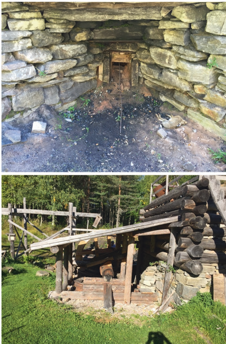
Fig. 6.4 Reconstruction of blast furnace for Bog ore at Lapphyttan from approximately year 1100 (Västmanland Archeology Board 2016 )
