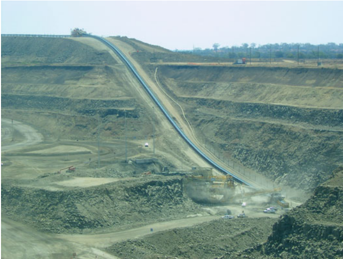
Fig. 7.21 Semi-mobile IPCC system in an Australian mine
