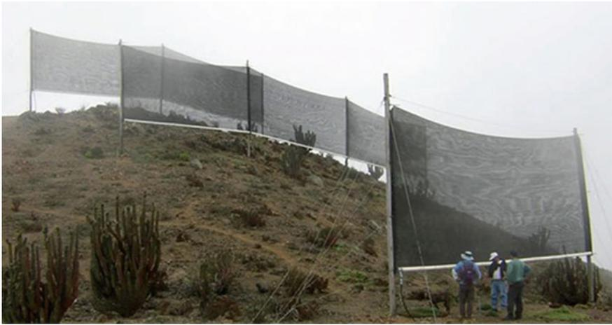
**Fig. 14.10** Fog collector system and community members in Falda Verde, Chañaral, Atacama (courtesy of *Cereceda P*, CDA—Centro del Desierto de Atacama)
