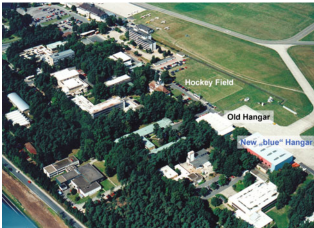
Fig. 9.3 New Hangar in Braunschweig for ATTAS
