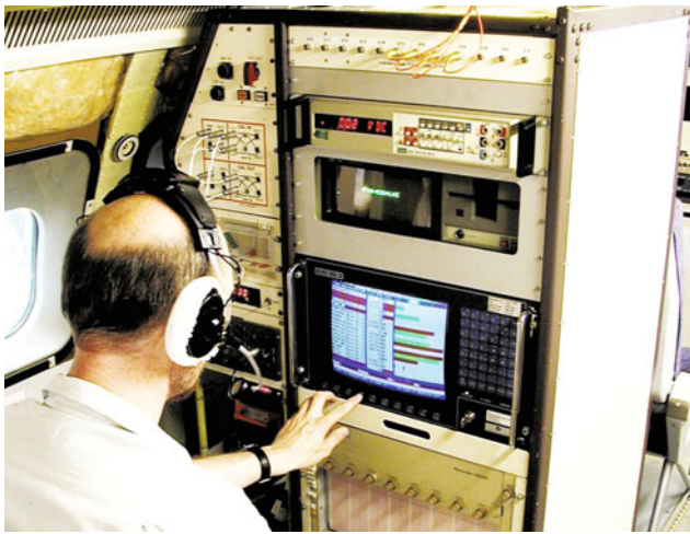
Fig. 9.22 Measurement system cabinet being operated by Adolf Zach
