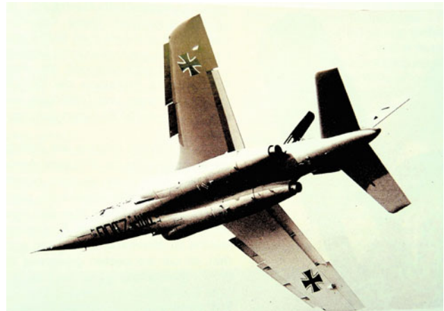
Fig. 6.125 TST test aircraft with deflected maneuvering slats and flaps
