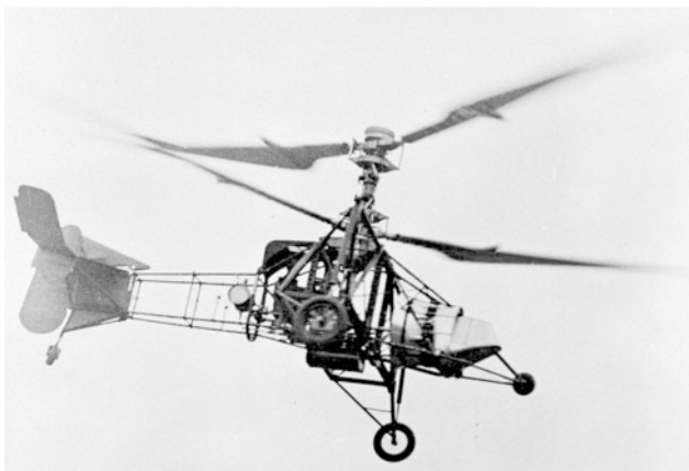
Fig. 2.13 Experimental helicopter Breguet-Durand Coaxial “Gyroplane Laboratoire” (1941), (Credit American Helicopter Society)
