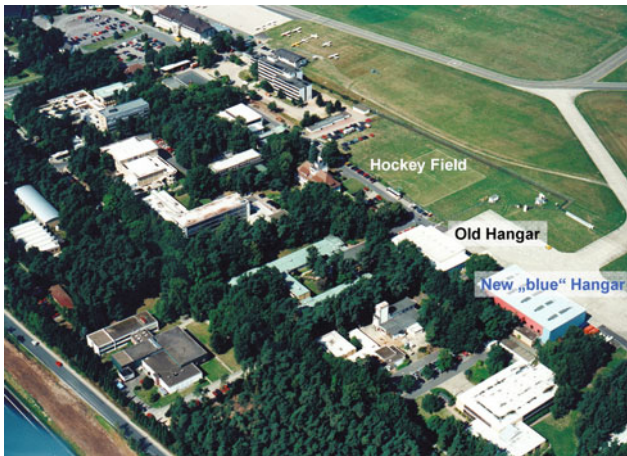
Fig. 9.3 New Hangar in Braunschweig for ATTAS
