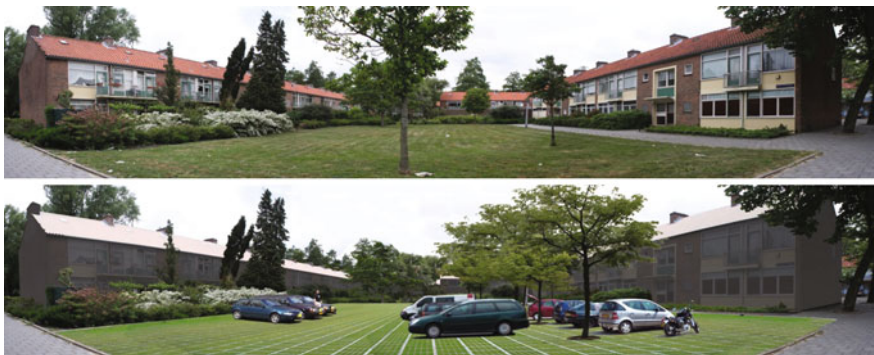
Fig. 20.3 Above Existing semi-public inner courtyard. Below Adaptation measures which improve thermal comfort and increase parking space are light roofs, middle-dark facades, additional trees and permeable pavement with grass
