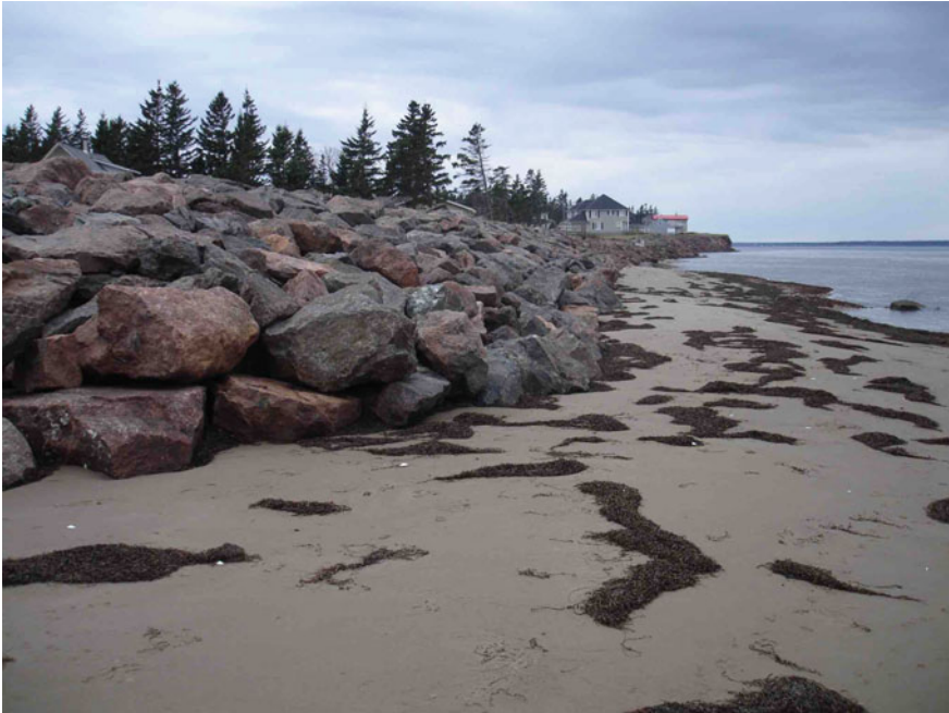
Fig. 5.2 Large rock riff-raff in the region of Pointe-du-Chêne
