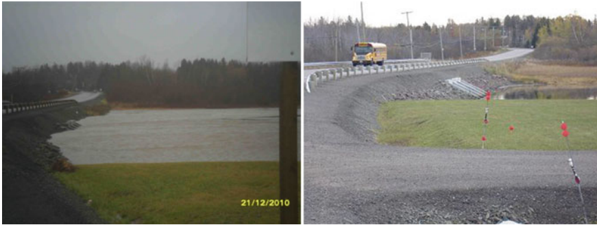
Fig. 5.5 The newly elevated bridge of Pointe-du-Chêne during the storm of 2010 and under normal conditions
