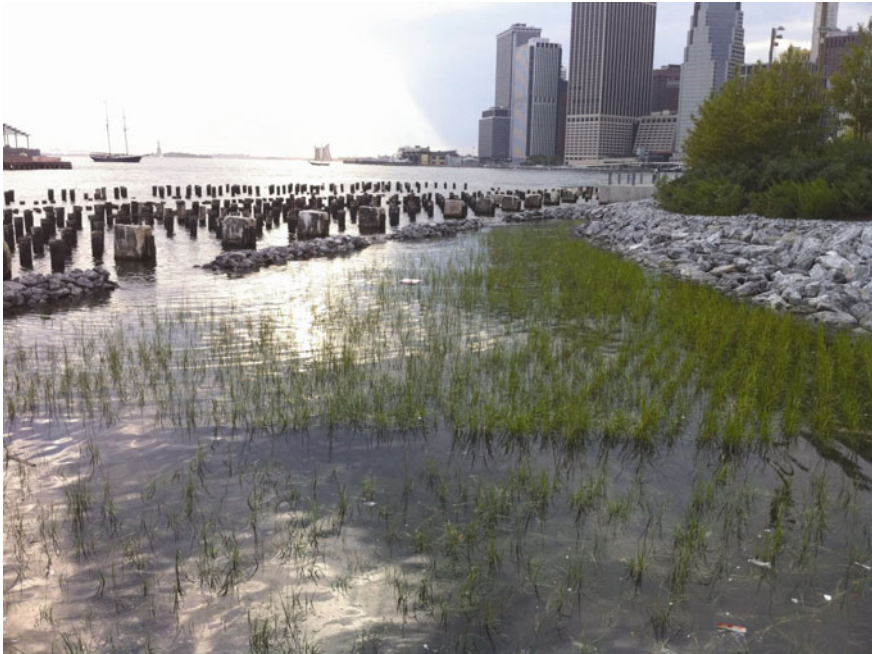
Fig. 13.3 Example of a living shoreline. Creating a soft edge shoreline, Brooklyn Bridge Park, New York City. Source Department of City Planning, City of New York City, 2011
