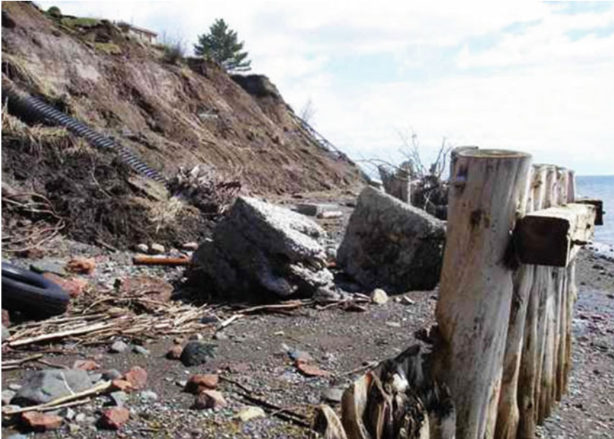
Fig. 5.4 Wood palisade with filling material in Carleton, Gaspé Peninsula
