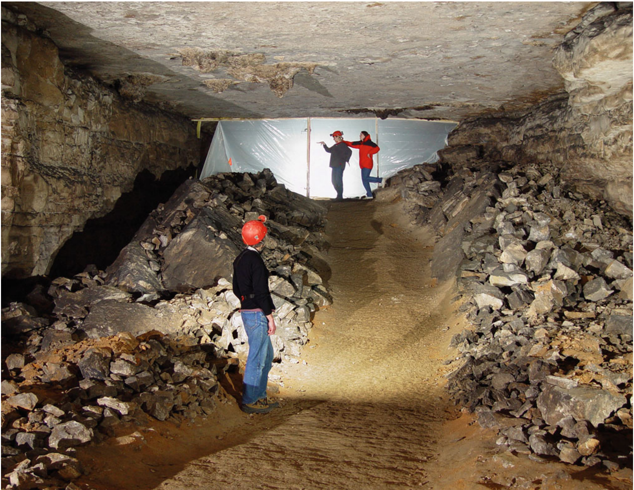
Fig. 10.8 This artificial wall of wood and plastic sheeting was installed in Gothic Avenue to block the flow of moist air toward Booth's Avenue. Condensation was greatly curtailed, but the wall was
