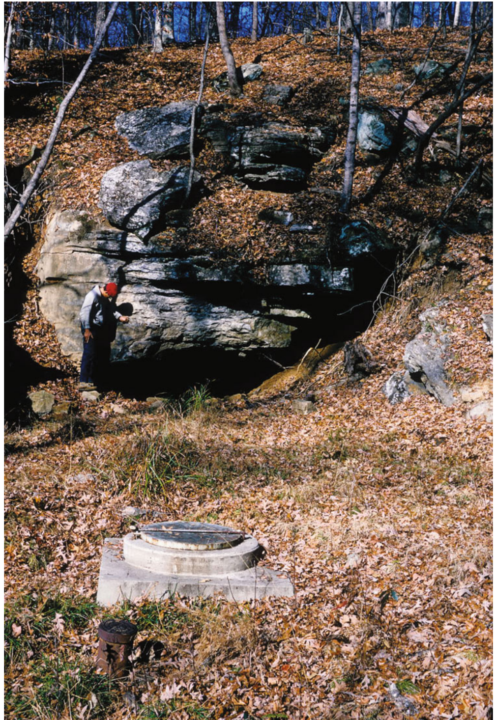
Fig. 8.9 Collins Spring on Flint Ridge. Like other of the Haney springs, Collins Spring has been capped and connected to a collector system to provide water for the Park. Photograph by the authors
