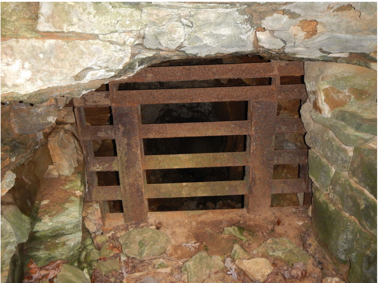
Fig. 17.5 Current bat-friendly angle iron steel gate installed in July 1994 at the entrance to Colossal Cave in Mammoth Cave National Park, Kentucky. NPS Photo
