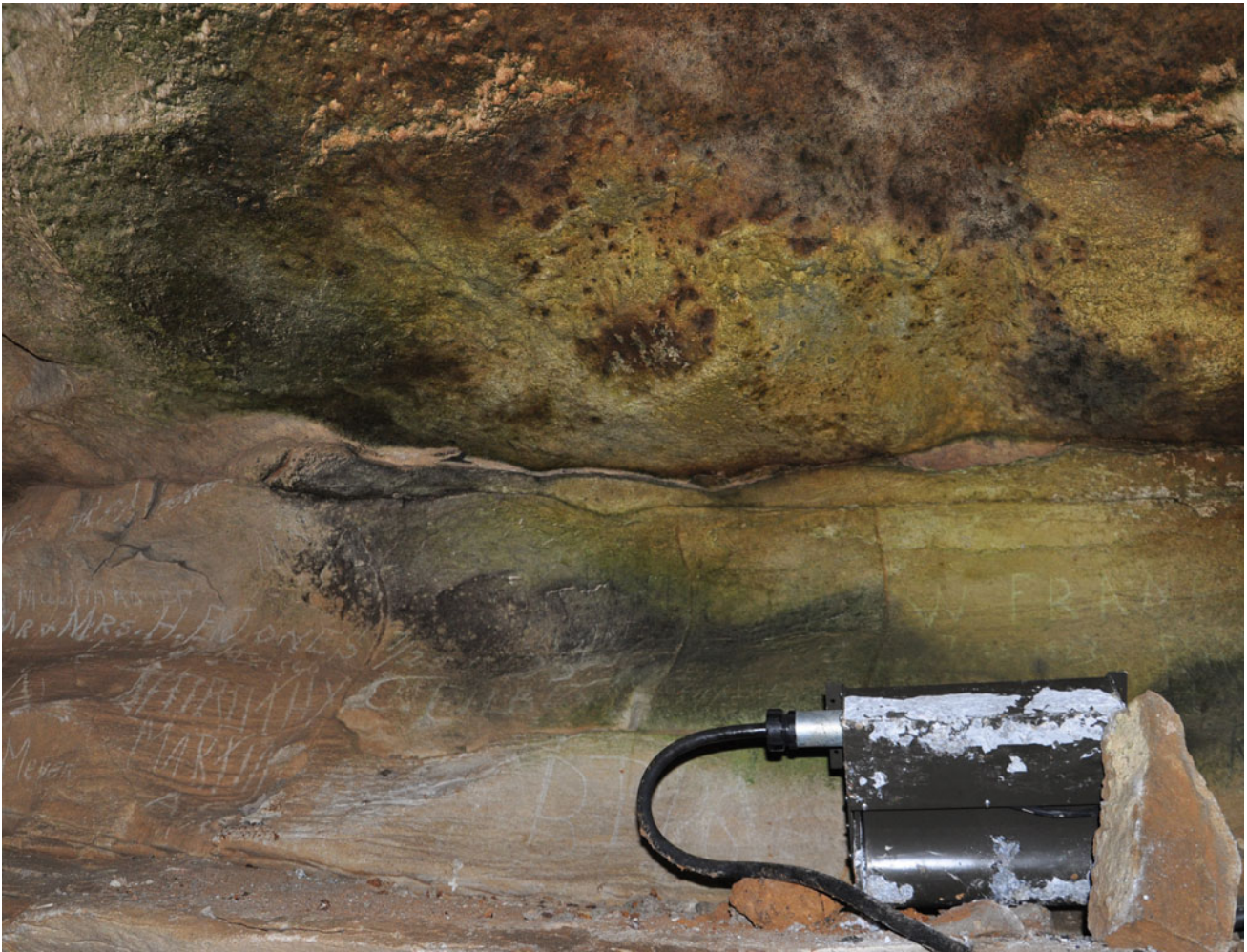
Fig. 18.6 Full spectrum lights installed as part of the new lighting system beginning in 2003 have resulted in continued significant lamp flora problems in Mammoth Cave. Brown material growing on the algae is mold. The $560 (in 2003) aluminum fixture lighting the area
